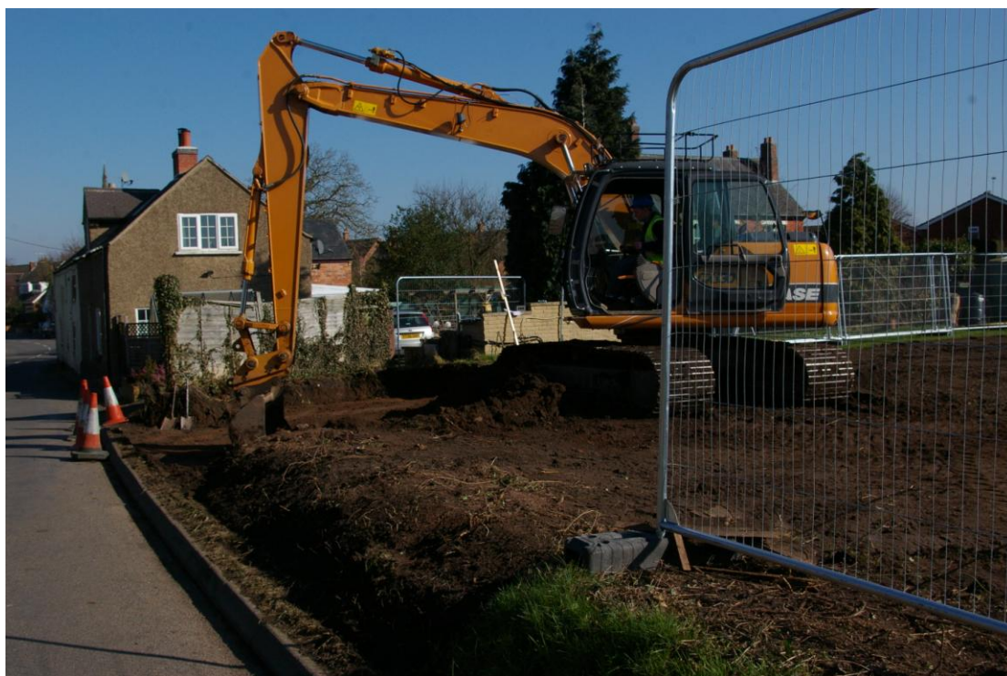
Plate 3: Work in progress at street frontage, looking north
