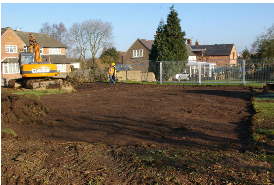
Plate 2: Grass area stripped of topsoil, looking north north-west
