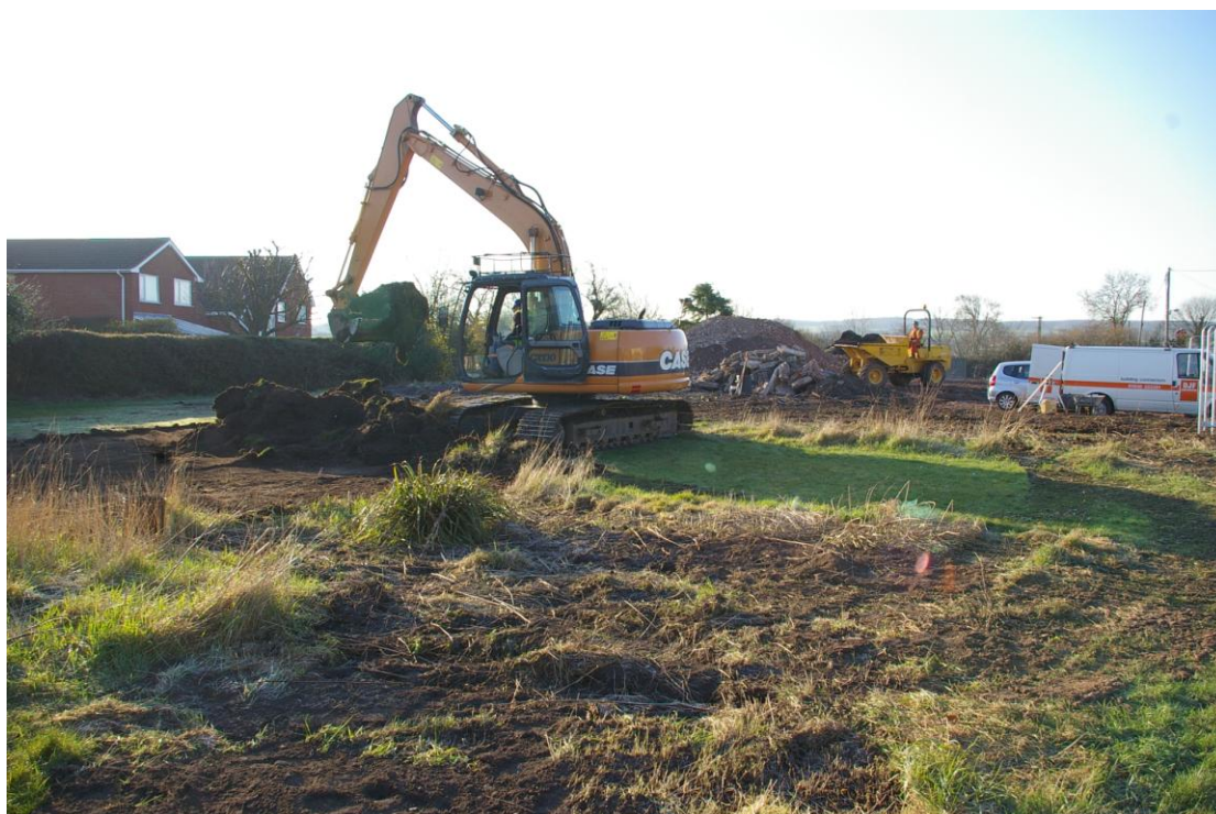
Plate 1: Work in progress stripping grass area, looking south-east
