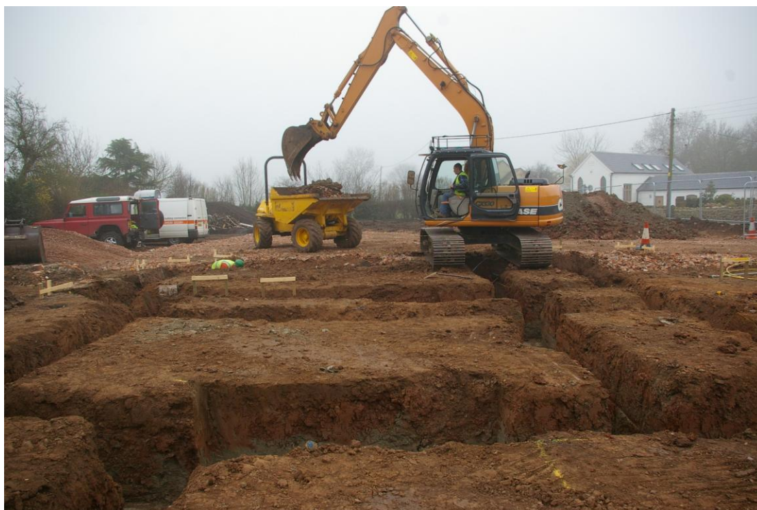
Plate 5: Work in progress on trenches in centre of site, looking south
