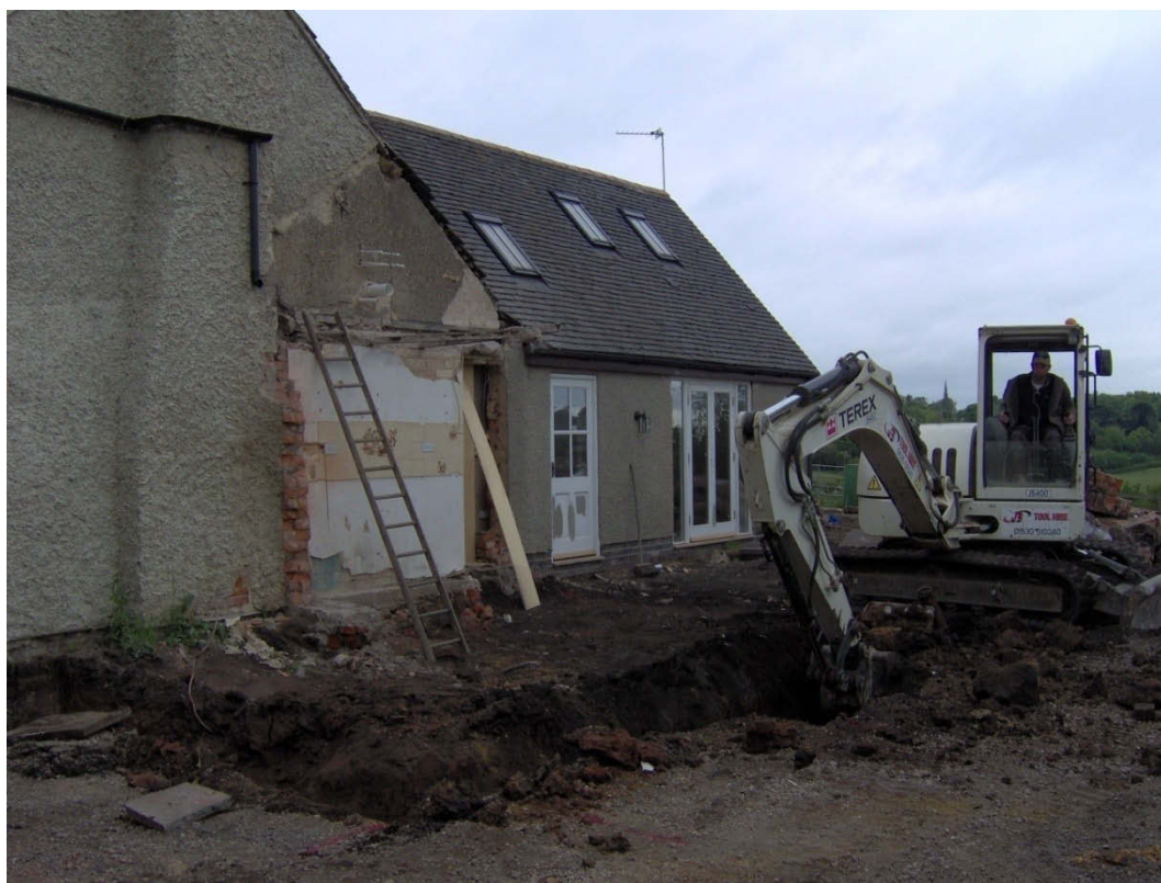
Figure 3: Excavation of the footings in progress, showing their position in relation to the house and the site of the former extension (now demolished). Looking north.
