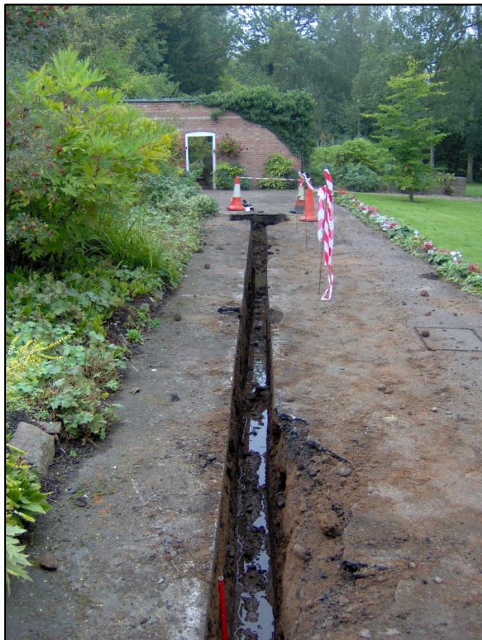
Plate 2. Drain Trench 1 looking east
