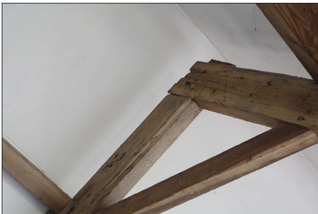
Figure 11 Collar and apex. LHS truss.
