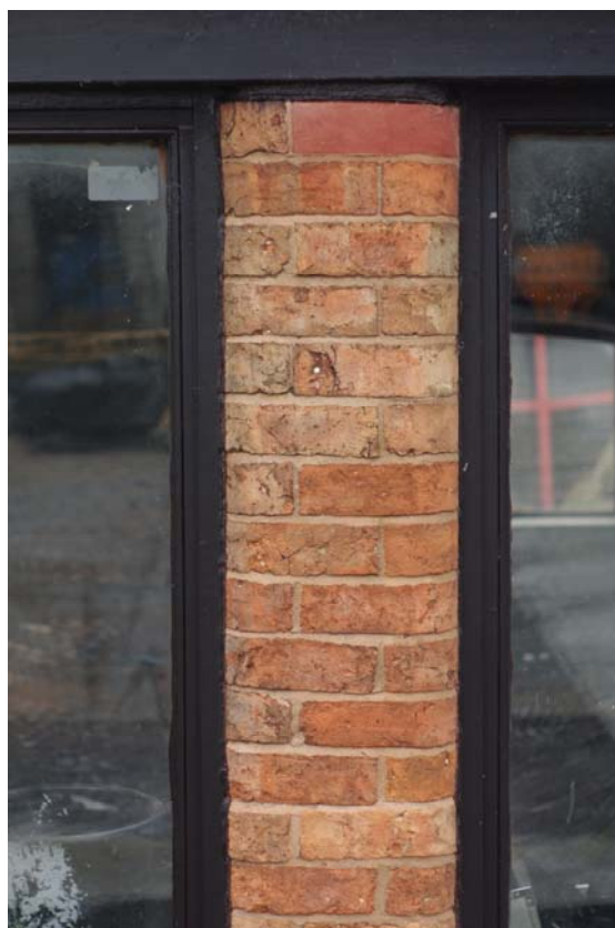
Figure 8 Pier at front showing bull-nose bricks
