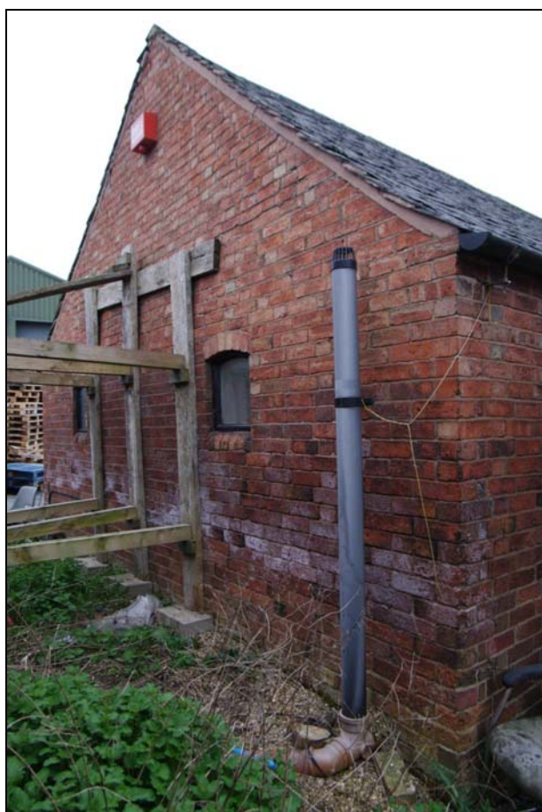
Figure 7 Right hand gable
