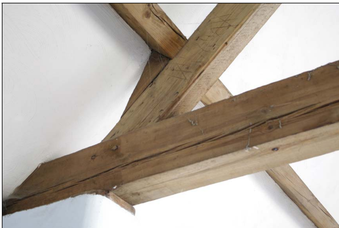
Figure 10 Junction of tie beam, principal and purlin. Rear of LHS truss
