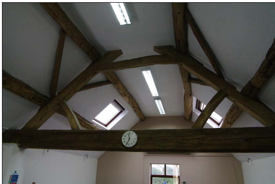
Figure 14 Roof structure of converted 18 th century barn
