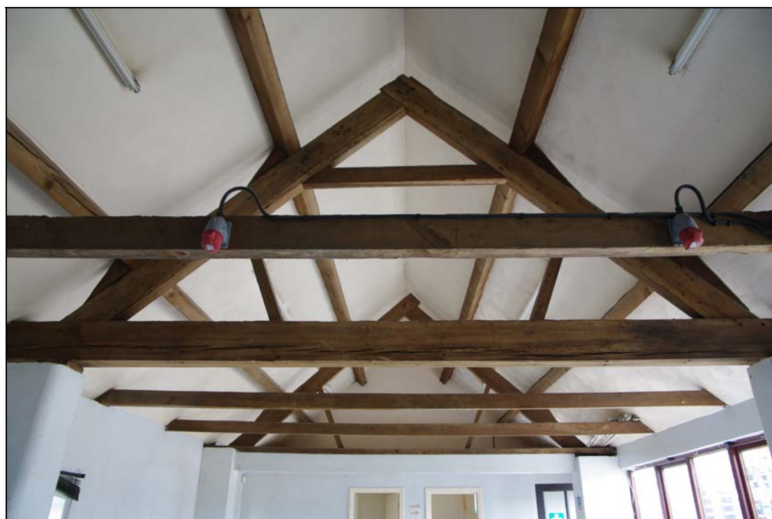
Figure 9 Roof structure. Looking to RHS
