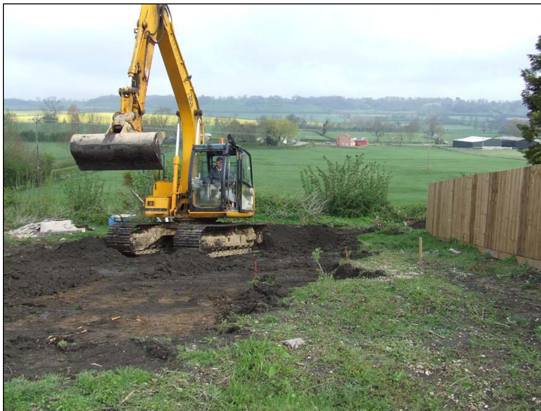
Figure 4 Topsoil stripping, looking north. Note earthworks in pasture to the rear.
