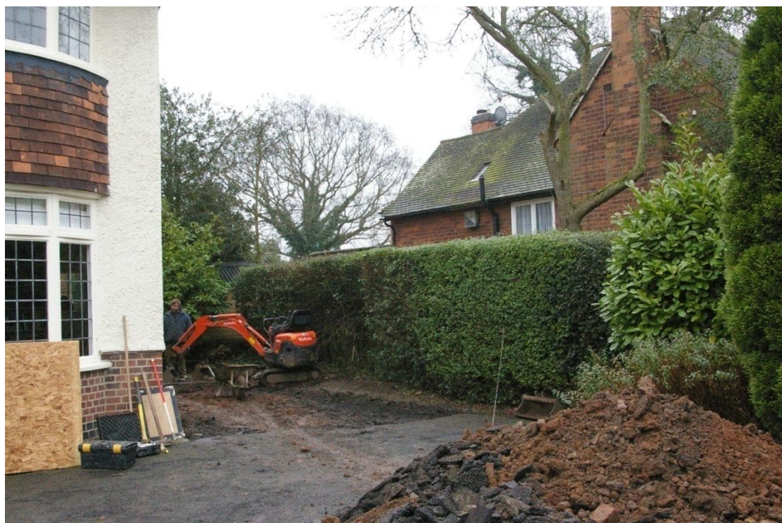
Plate 1: Machine excavating foundation trenches for the new extension
