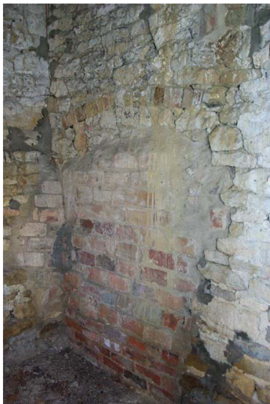
Figure 10 Blocking seen from inside the barn. Looking south-west.
