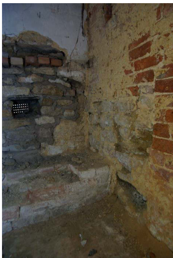
Figure 16 Looking north-west. Stonework at base of wall
