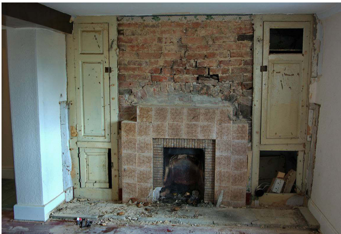
Figure 7 Dining Room looking east.
