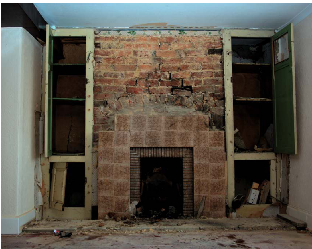
Figure 8 Dining room looking east
