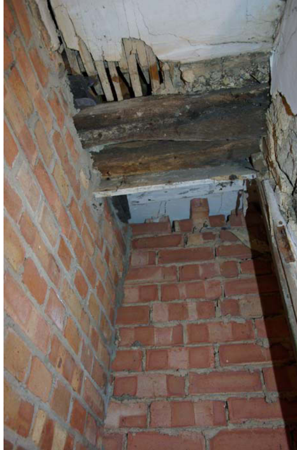
Figure 14 Looking east. Doorframe to right hand side and above; beams over
