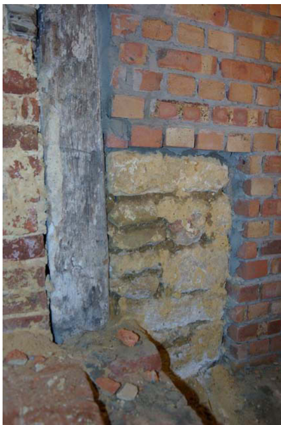
Figure 15 Looking north. Post, plinth, stonework and modern brickwork over.
