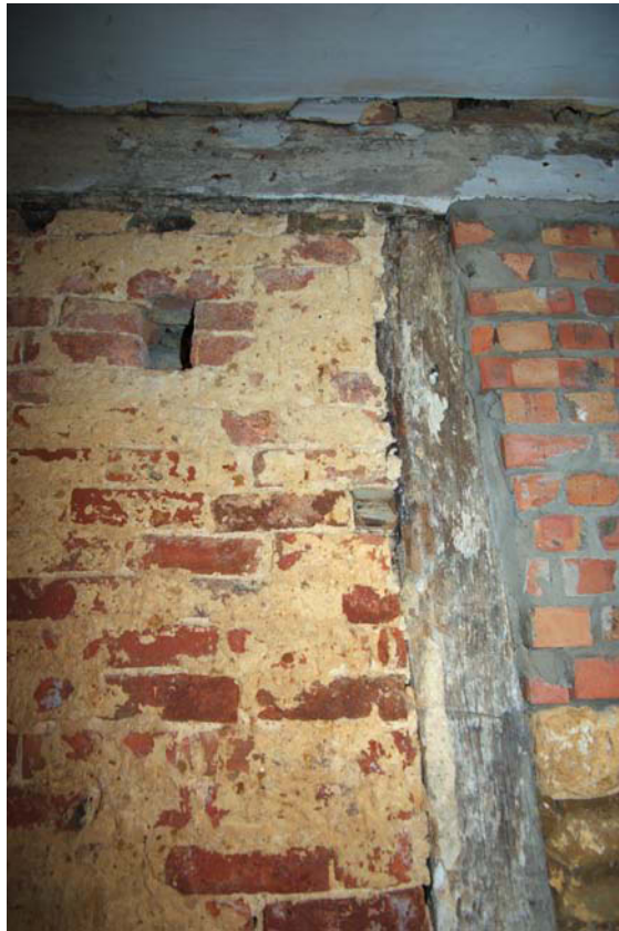
Figure 12 Note chamfered beam running over post, modern brick to the right hand side with stone under; earlier brick panelling to left hand side with aperture, and sawn-off shelf bracket against post.
