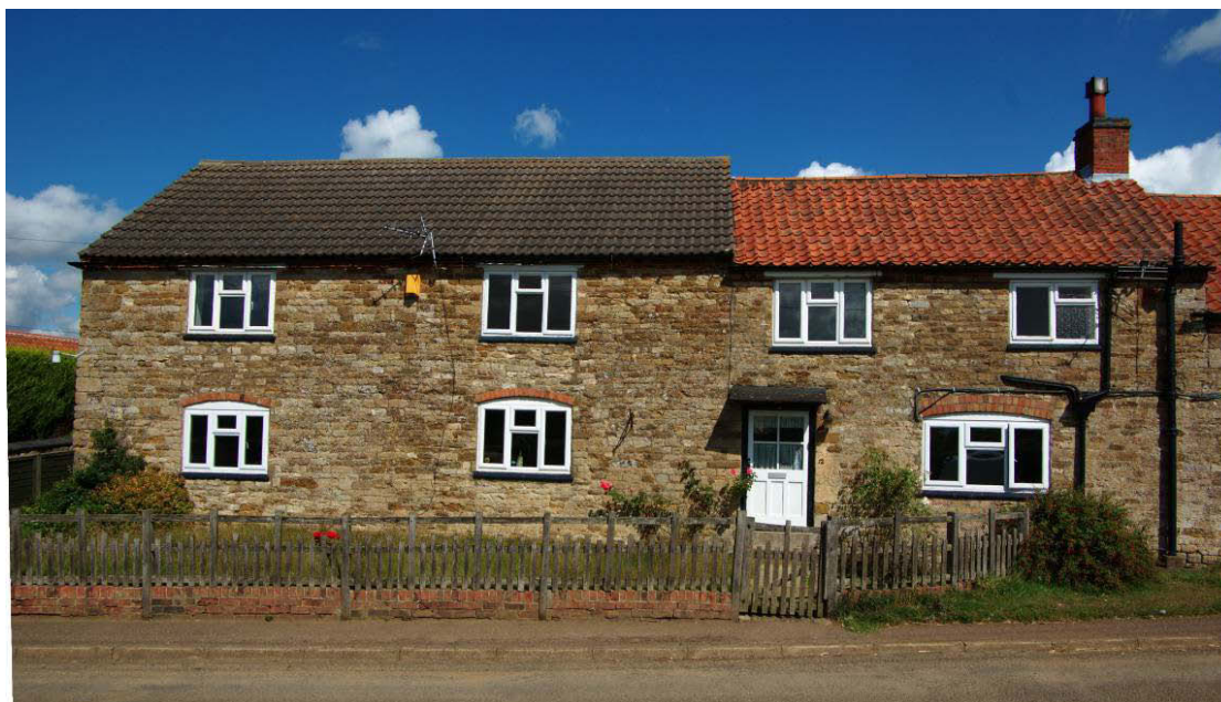
Figure 4 Frontage, west and east units. Looking north.
