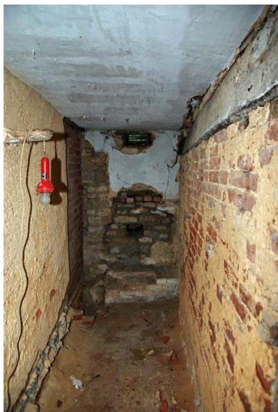
Figure 11 Passage, looking west. Note modern wall blocking opening to rear left hand side; overhead beam and brick panelling to right hand side; stone exterior wall to rear with modern vents.
