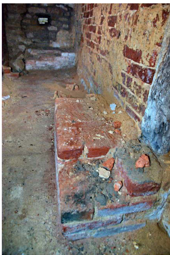
Figure 18 Looking west. Plinths
