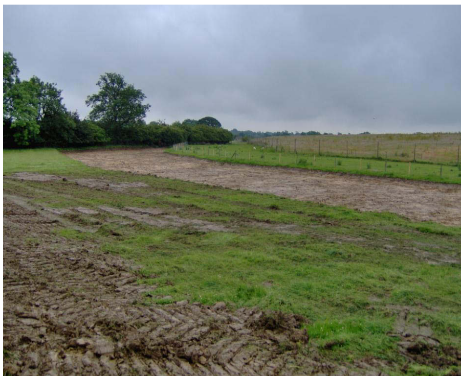
Figure 11 Phase 8 showing stripped haul road
