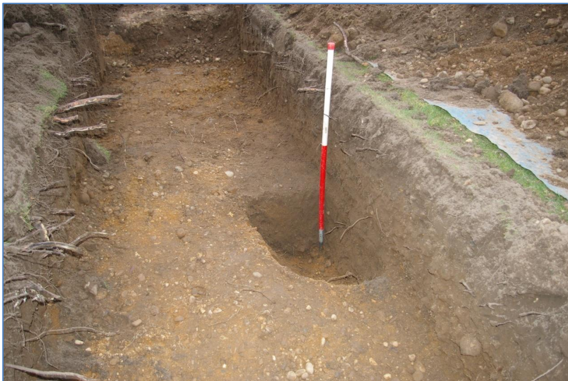
Figure 6 Trench 2, looking south-east. Pit [2], and in the background, a concrete wall footing
