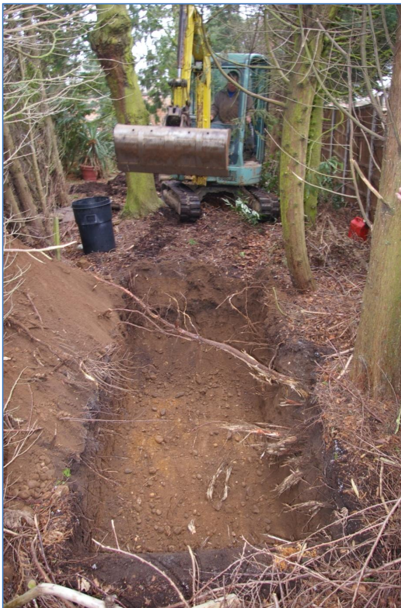
Figure 4 Trench 1(E) under excavation, looking west.
