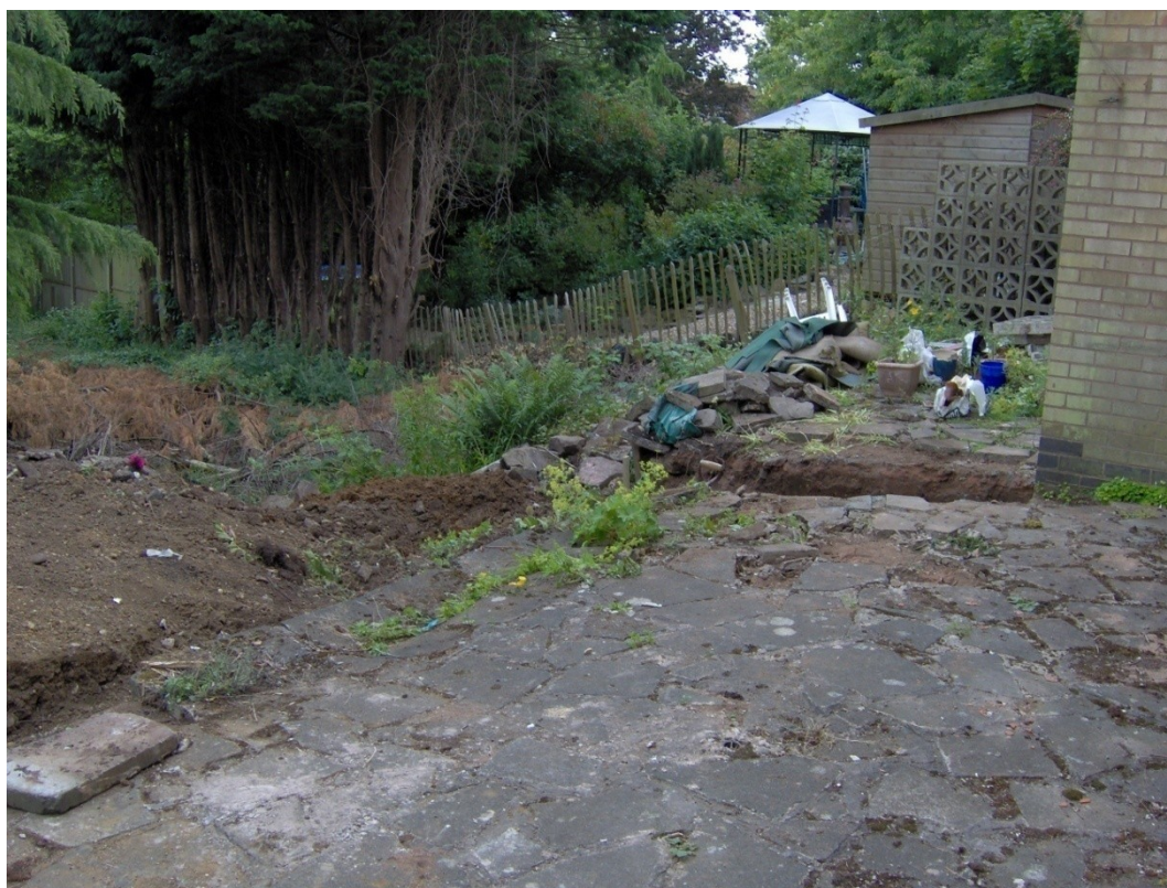
Figure 5: Ground to the rear of no. 11 dropping down into the old quarry workings – looking south-east
