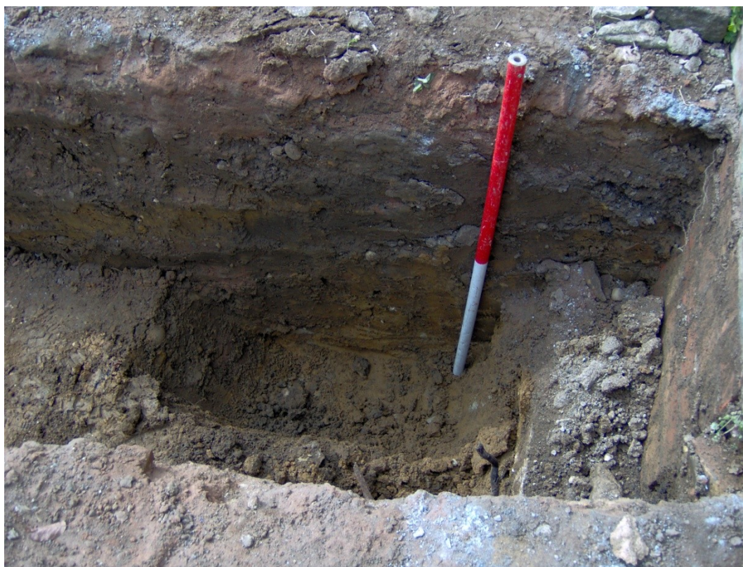
Figure 4: The southern rear footing showing the quarry edge dropping away (to the left of the scale) – looking south
