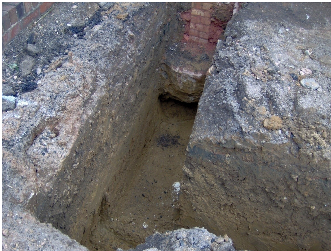
Figure 3: The northern front footing – looking north-east
