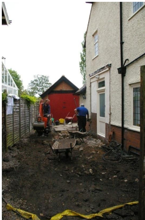
Plate 1: Ground clearance for the north gable extension
