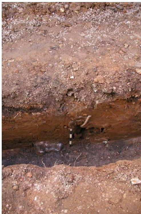
Plate 2: Granite stone and red clay spread within the Phase 2 extension foundation trenches (Looking north)
