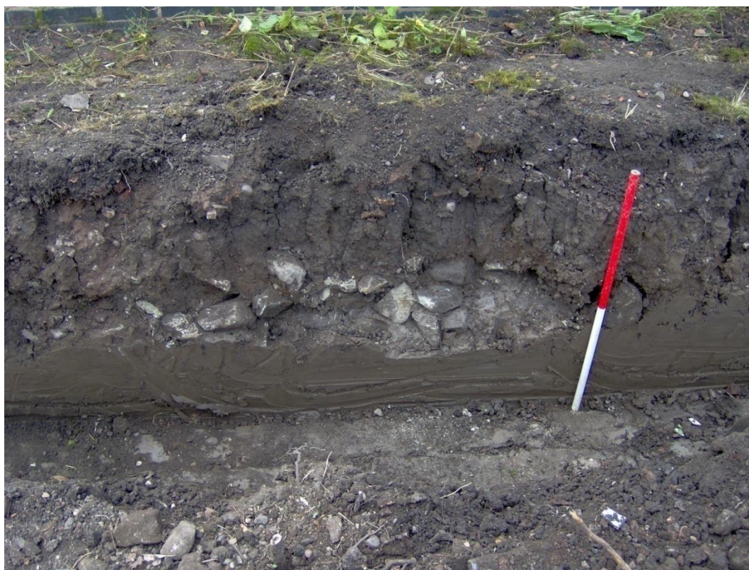
Figure 5: The western footing, looking west, showing stonework (4) resting on the natural clay (5)
