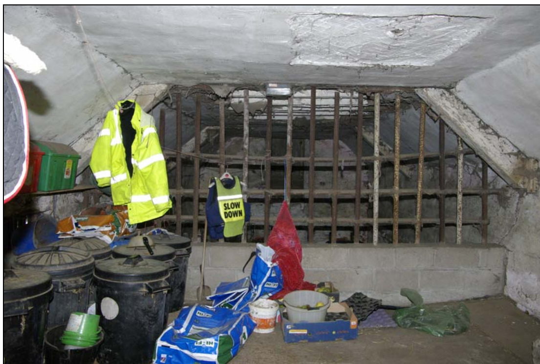
Plate 16. Range B, hayloft located within the eaves of three-bay stable block, with collared roof truss. Looking east.
