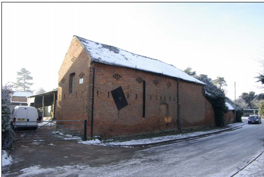
Plate 1. Range A, Barn 2 Church Lane elevation, looking south-west.
