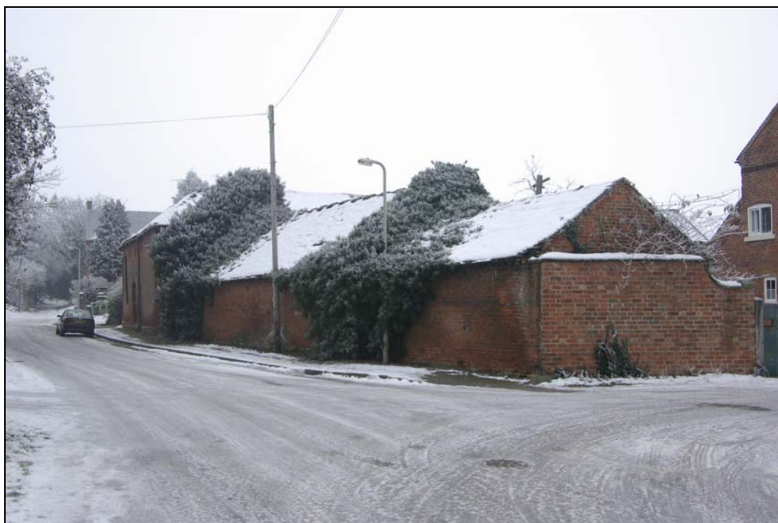
Plate 2. Range A, cowshed, looking south-east.
