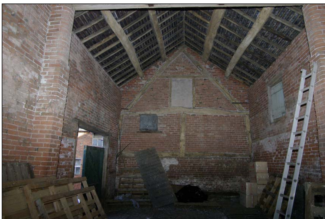
Plate 8. Timber cross-frame of 17th century box-framed structure. Looking north, with a change in the brick work on left-hand side indicating the raising of the height of the roof.
