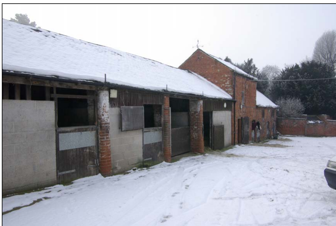
Plate 15. Range B, converted cow-shed. Looking south-west.
