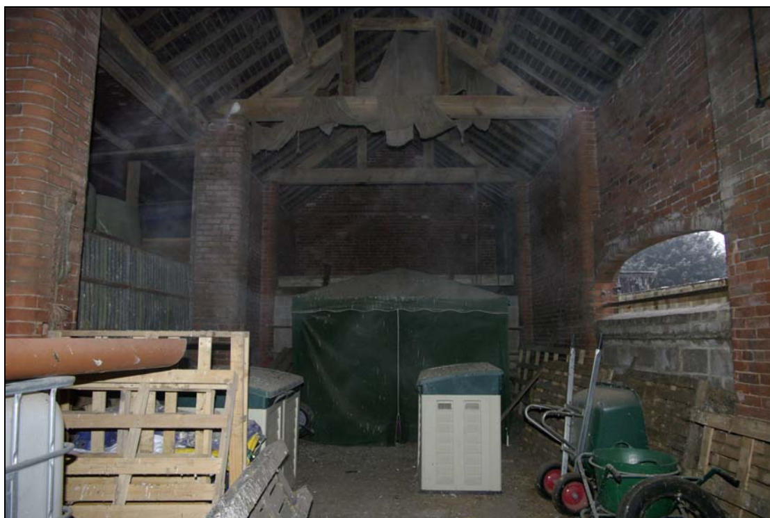
Plate 9. Range A, Barn 1 interior, with bolted, queen-post roof trusses. Looking south.
