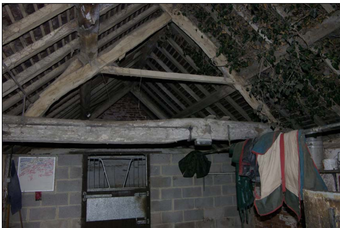
Plate 10. Range A, cowshed interior, with 18th century, pegged collar roof truss. Looking west.
