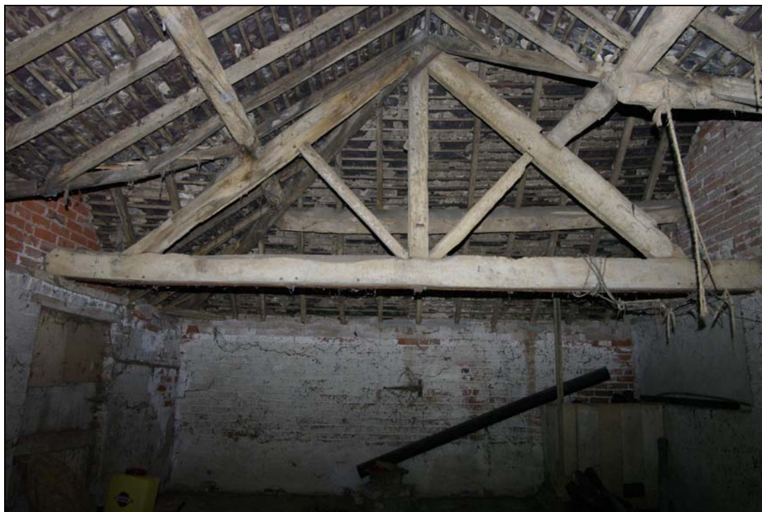
Plate 13. King-post roof truss over rebuilt central store. Looking north.
