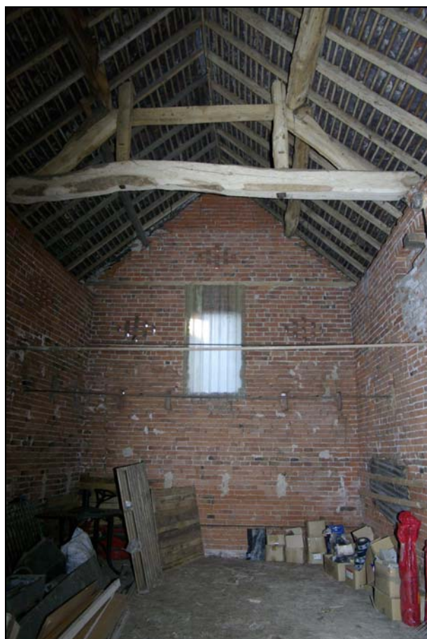
Plate 11. Range A, Barn 2 with queen-post roof truss. Looking east.
