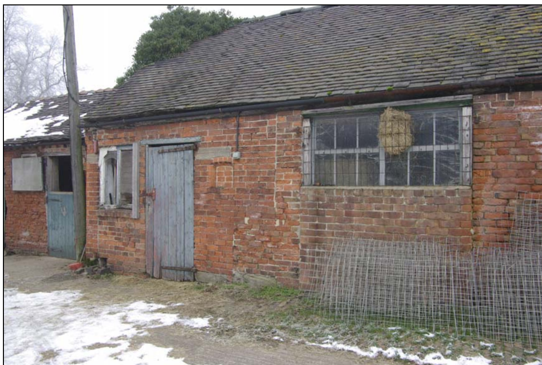
Plate 7. Range A, cowshed, with blocked and inserted openings. Looking north-west.
