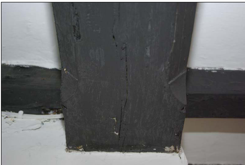
Plate 8. Late C17th chamfered and stopped axial beam, with decorative notching. Looking north-east.
