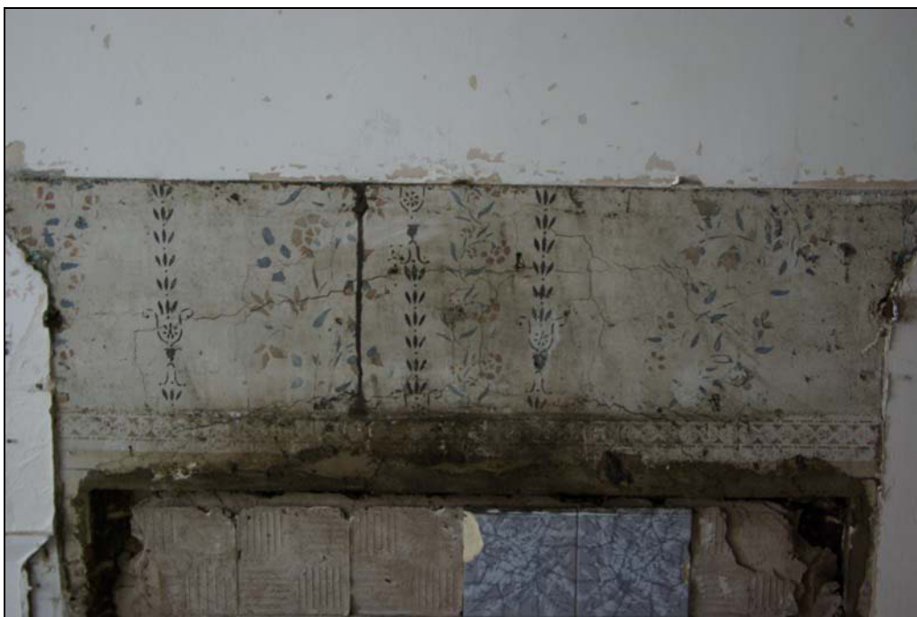
Plate 16. Painted plasterwork to late C18th chimney-breast. Looking south-west.
