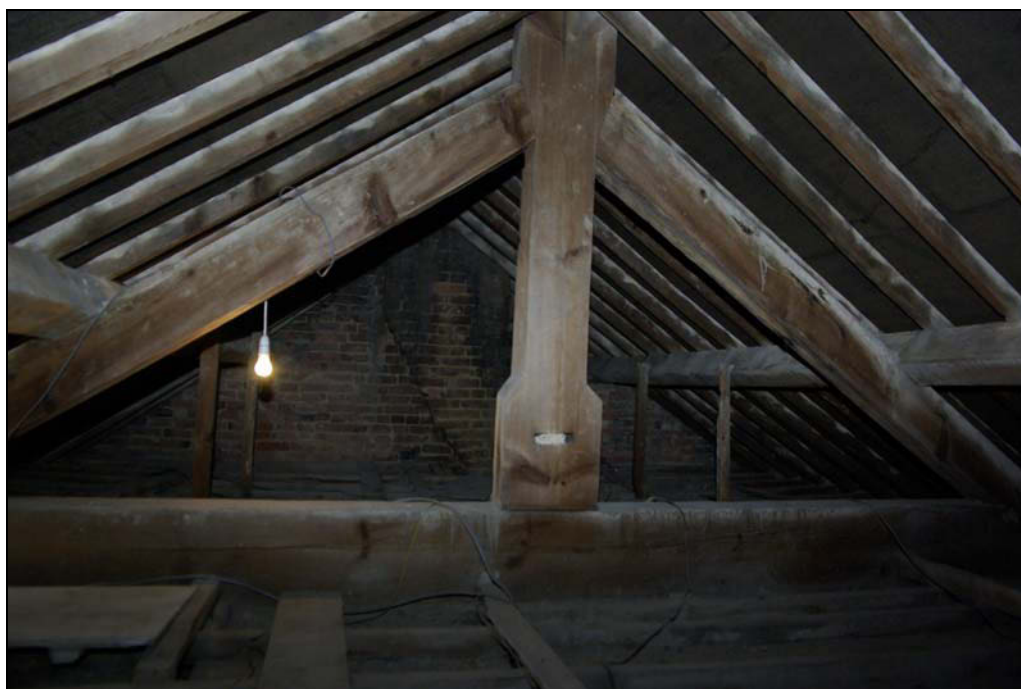
Plate 19. King-post roof truss within 1850+ range.
