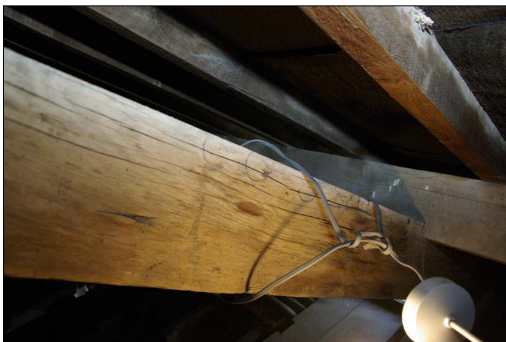
Plate 20. Shipping marks on imported Baltic timber of roof truss above.
