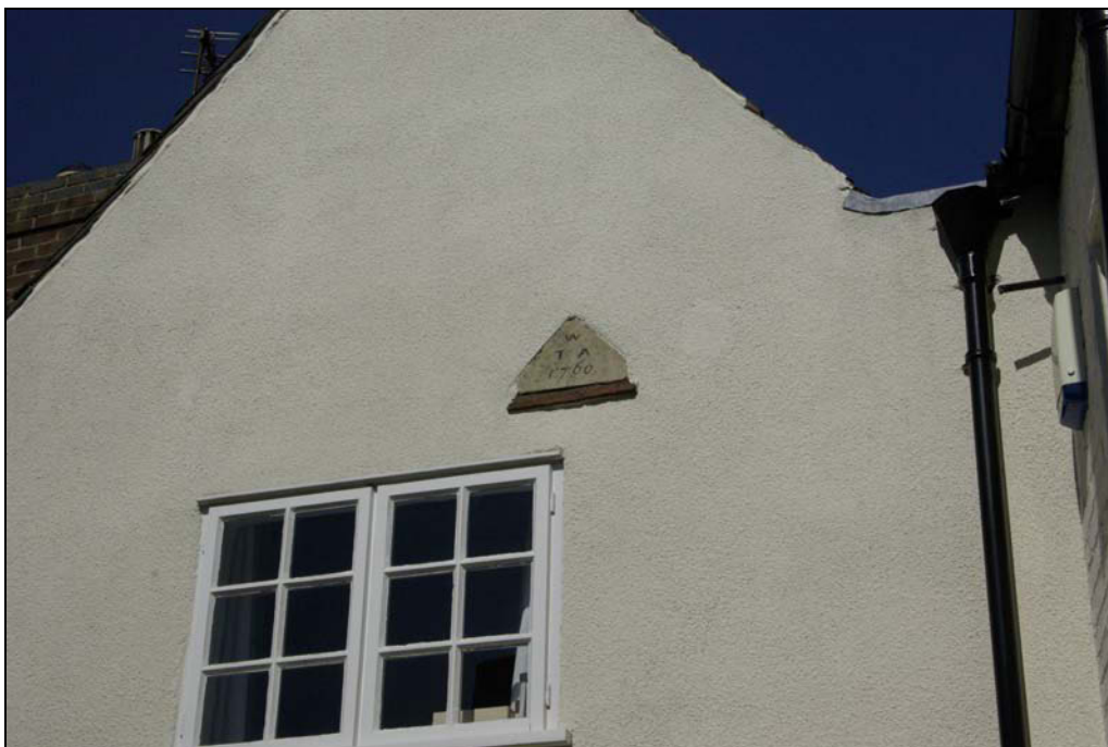
Plate 15. Re-sited datestone reading 'T.A.W. 1760'. Looking north-east.
