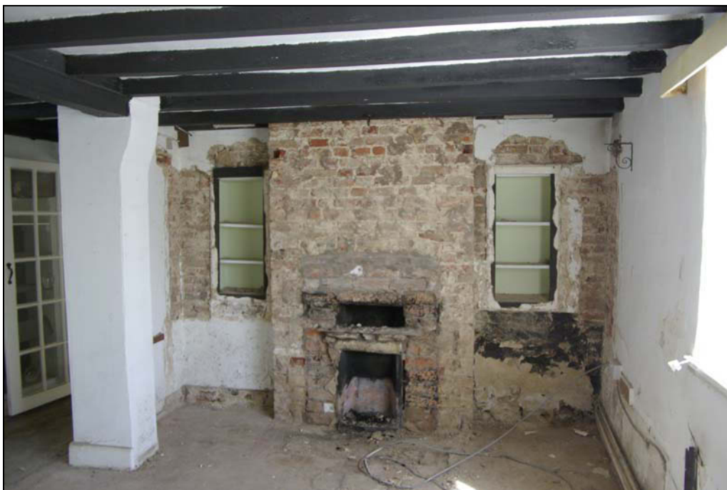
Plate 7. Position of ingle-nook. Late C17th axial beam, supported on 18th brick pier. C18th brick stack and spice cupboards. Looking north-east.
