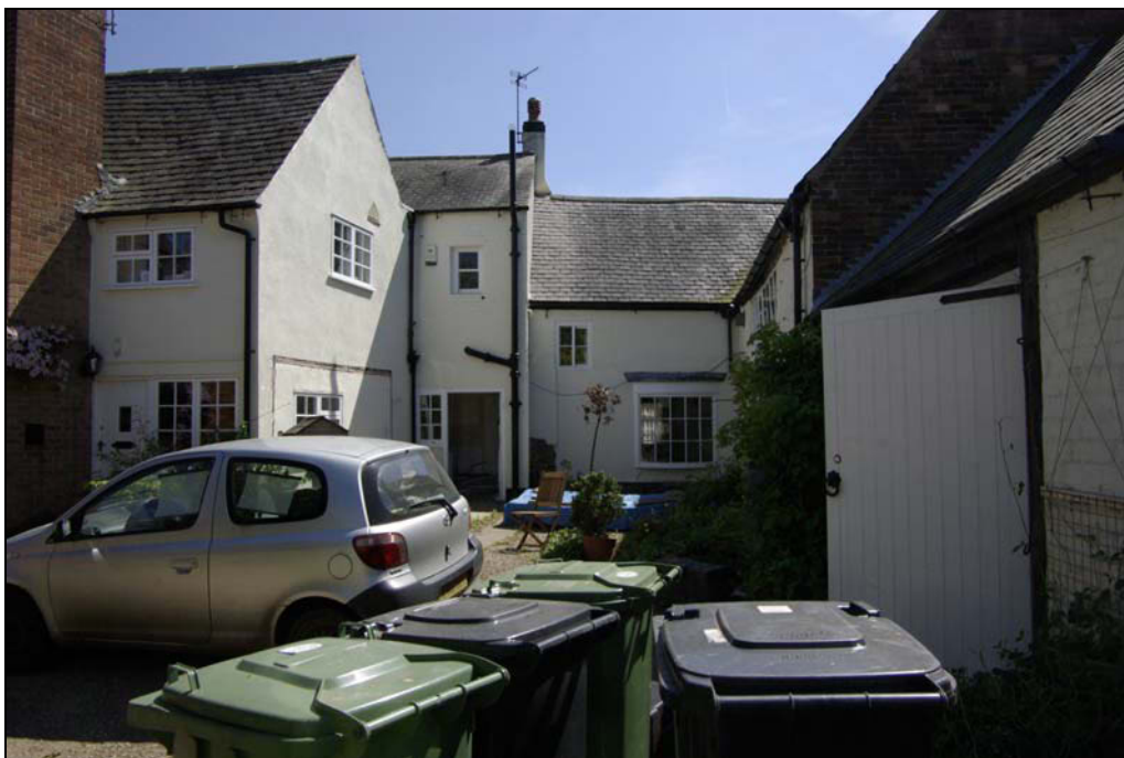
Plate 3. 15 Main Street, rear yard, looking south-east.
