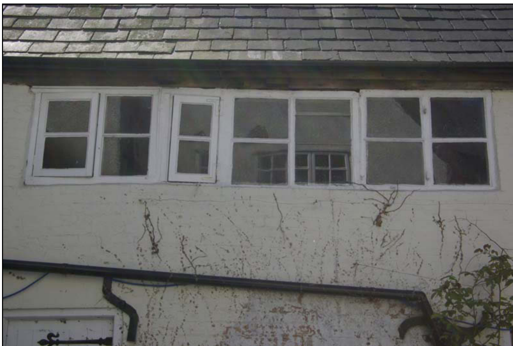
Plate 5. C18th first floor workshop window, looking south-west.
