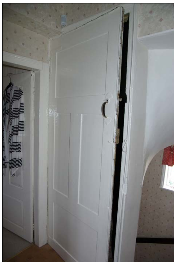
Plate 12. 18th century four-panel door, 1st floor. Looking east.
