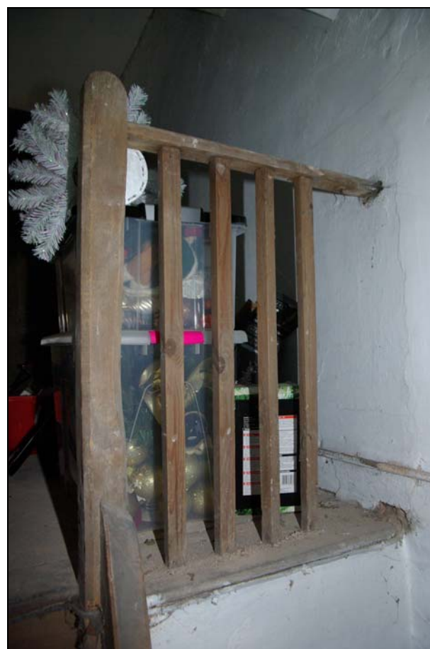
Plate 13. 18th century balustrade, 2nd floor. Looking west.
