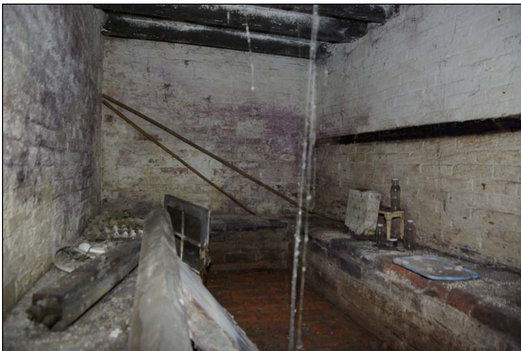
Plate 6. Cellar beneath sitting room, looking west.
