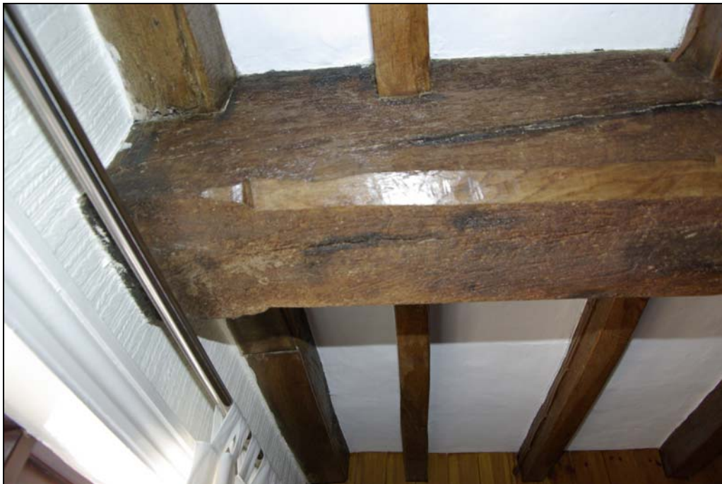
Plate 10. Chamfered and stopped transverse ceiling beam above northern bedroom. Looking north.
