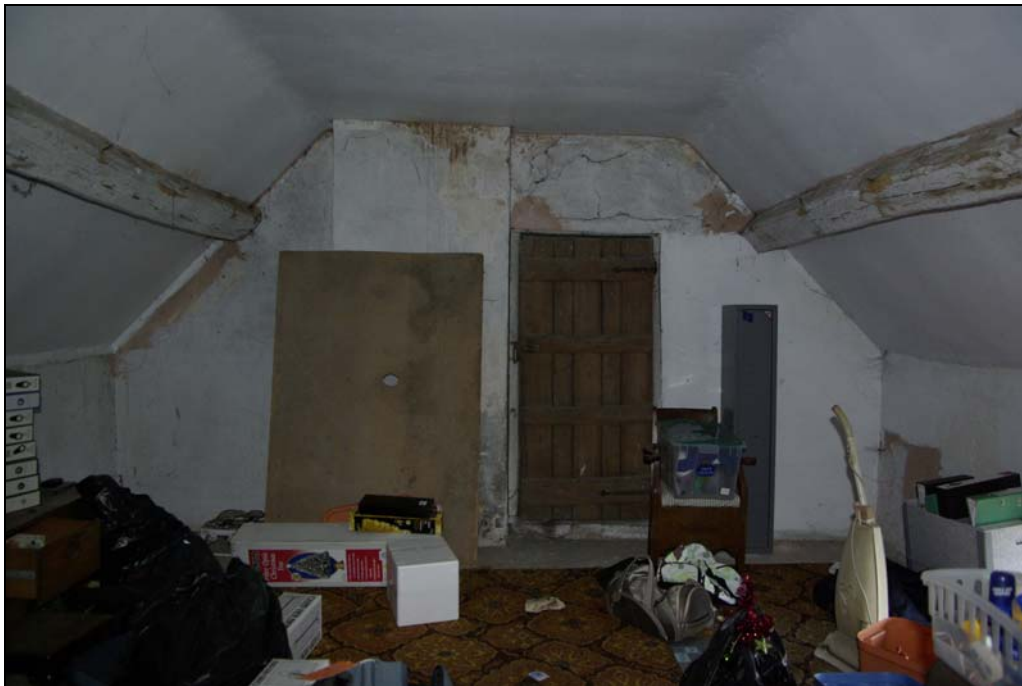
Plate 14. Northern attic room, looking north.
