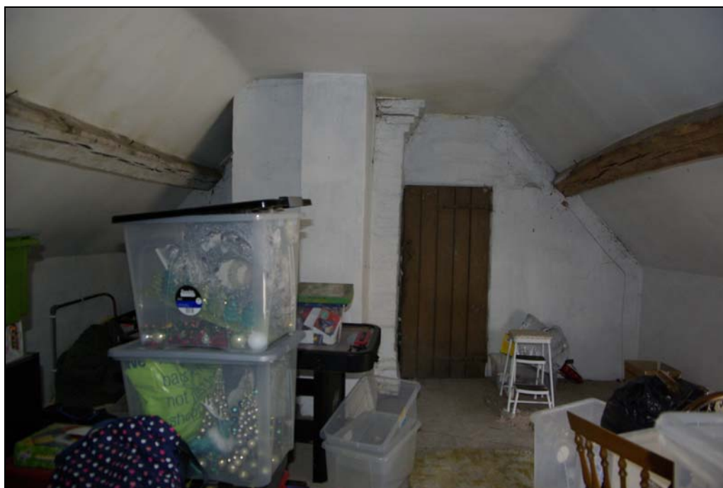
Plate 16. Central attic room, looking south.
