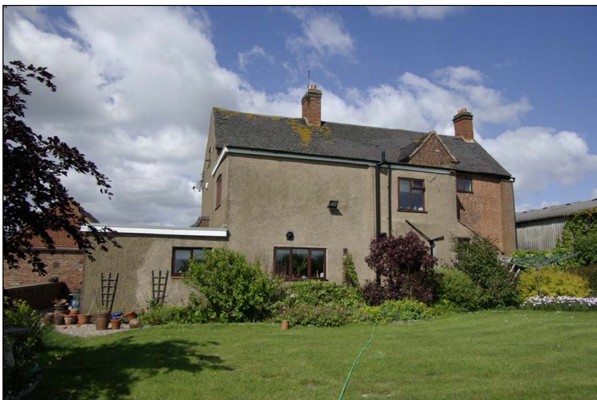
Plate 4. Rear elevation, looking west.
