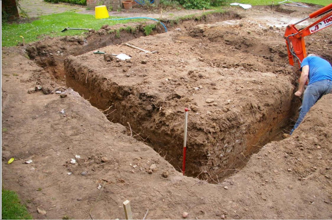
Figure 5: Footings being excavated in the south-west of the site, showing occasional outcrops of solid bedrock (foreground).
