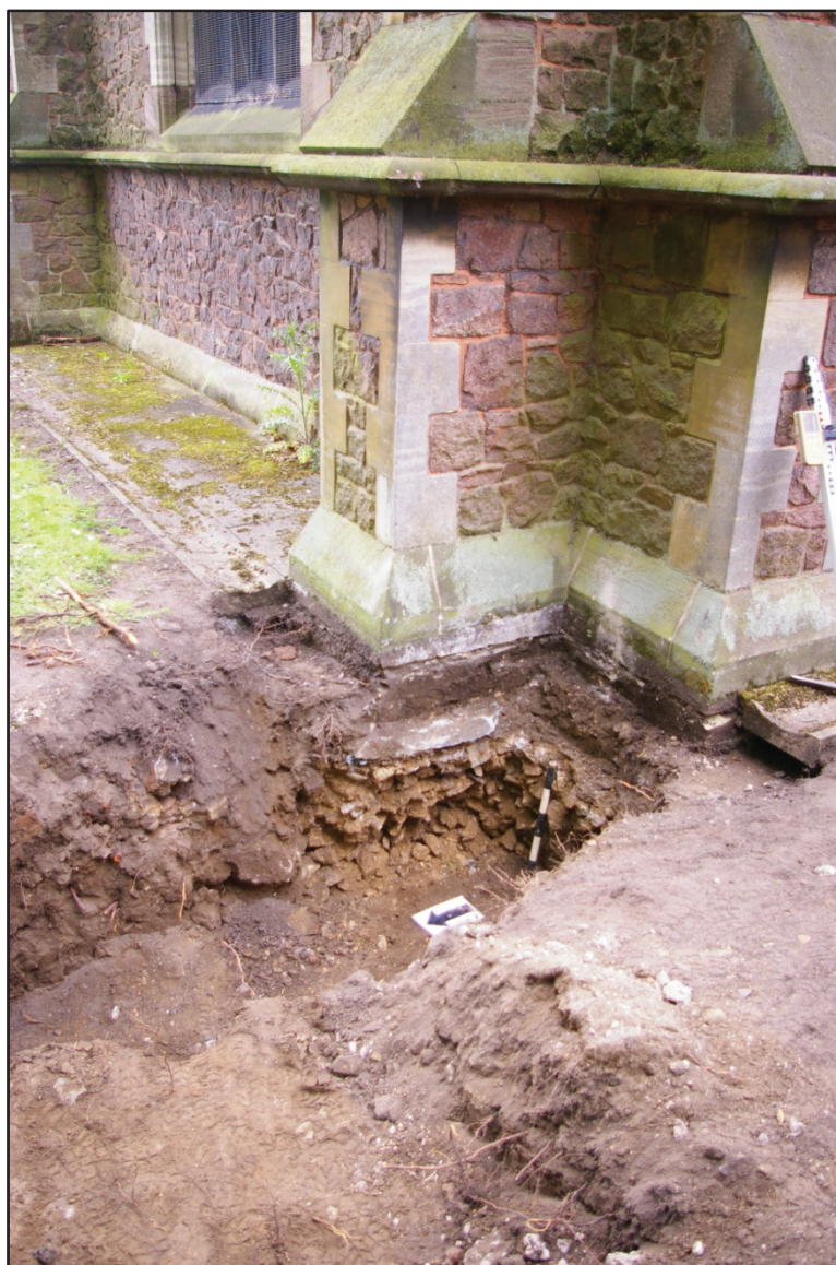
Plate 1. North Transept Foundations
