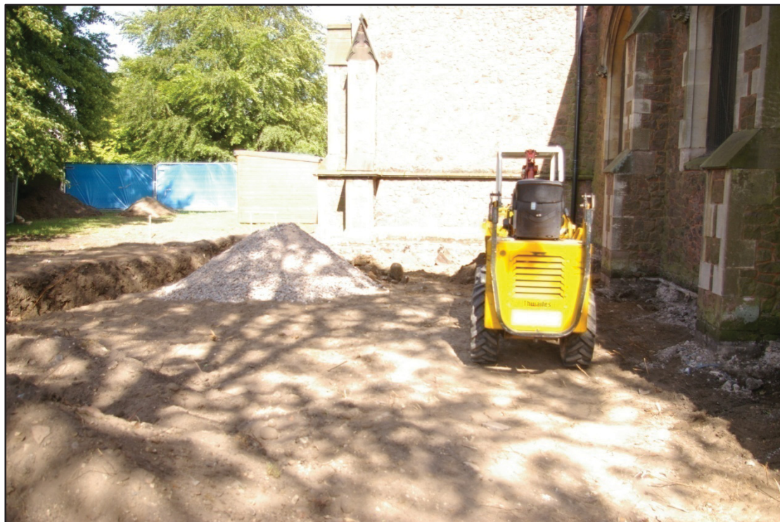
Plate 2. Area Strip and North Aisle foundations exposed
