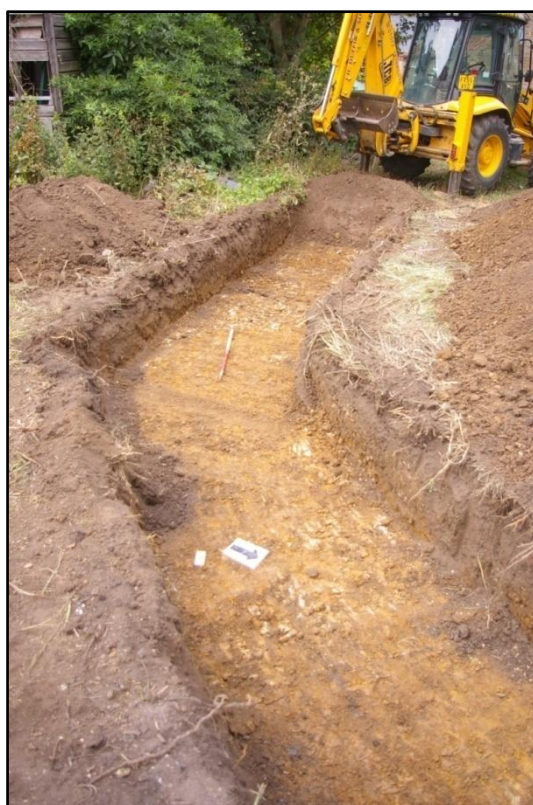
Plate 2 Trench 2 looking south-west
