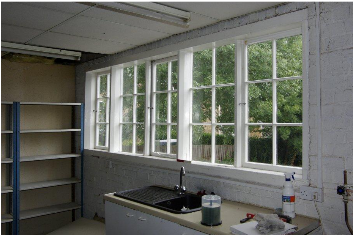
Figure 9 Middle window, first floor (023-024).
