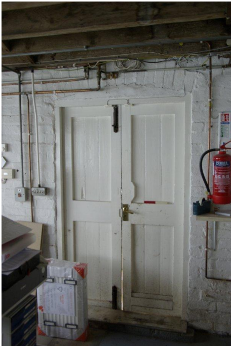
Figure 13 Door to be blocked during proposed works (047-048).
