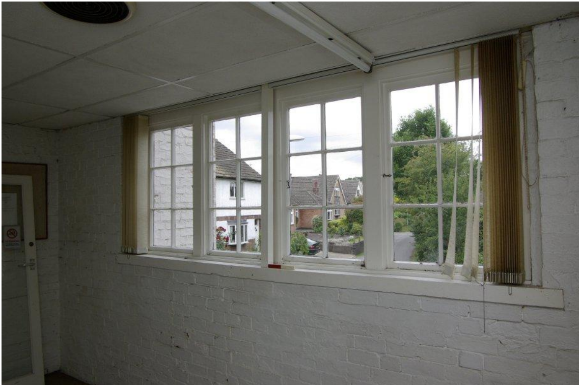
Figure 11 Window in west gable, first floor (039-040).
