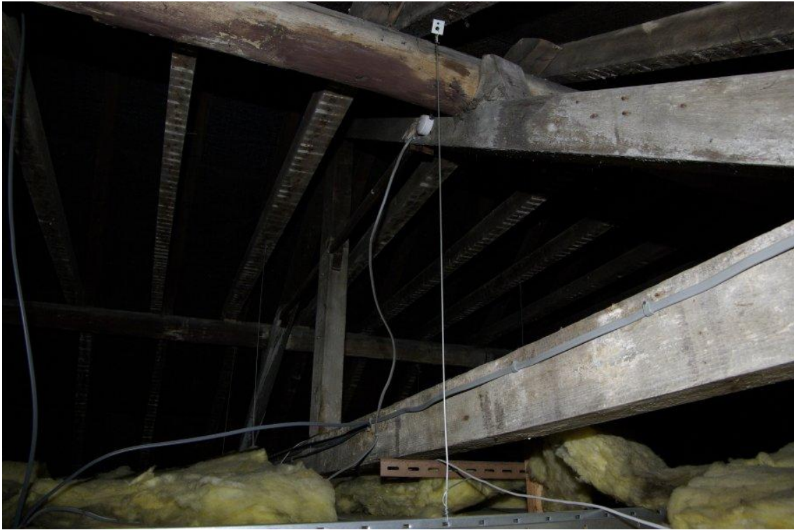
Figure 12 Limited view of roof structure (027-028).
