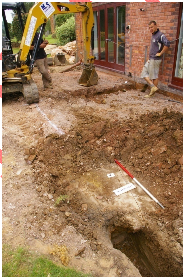
Figure 4 Modern concrete footings in easternmost end of trench (looking east).
