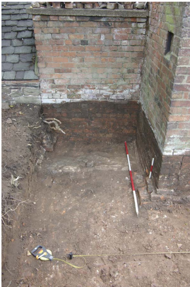
Photo 3. Granite sett surface (04) and offset brick footing (06) to 1858 cottage range.
