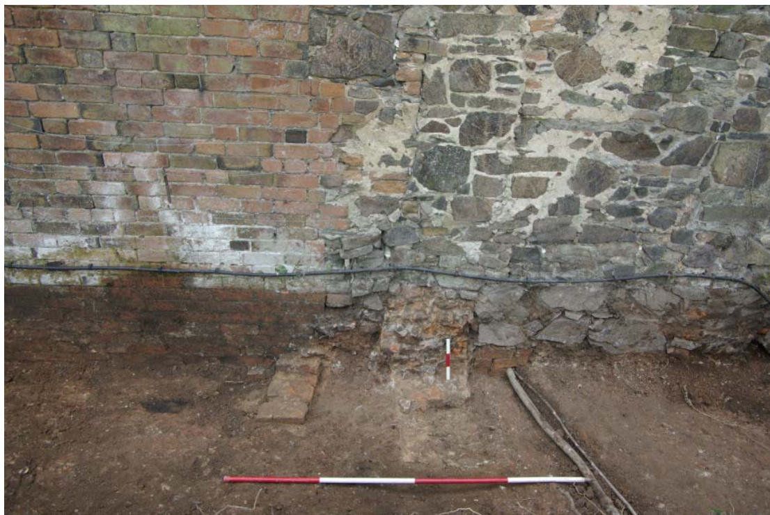
Photo 2. The vertical 30cm photo scale is resting on wall foundation (01), with foundation (02) to the left of this and lead water pipes to the right. The 2m photo scale is lying on cut feature (03).
