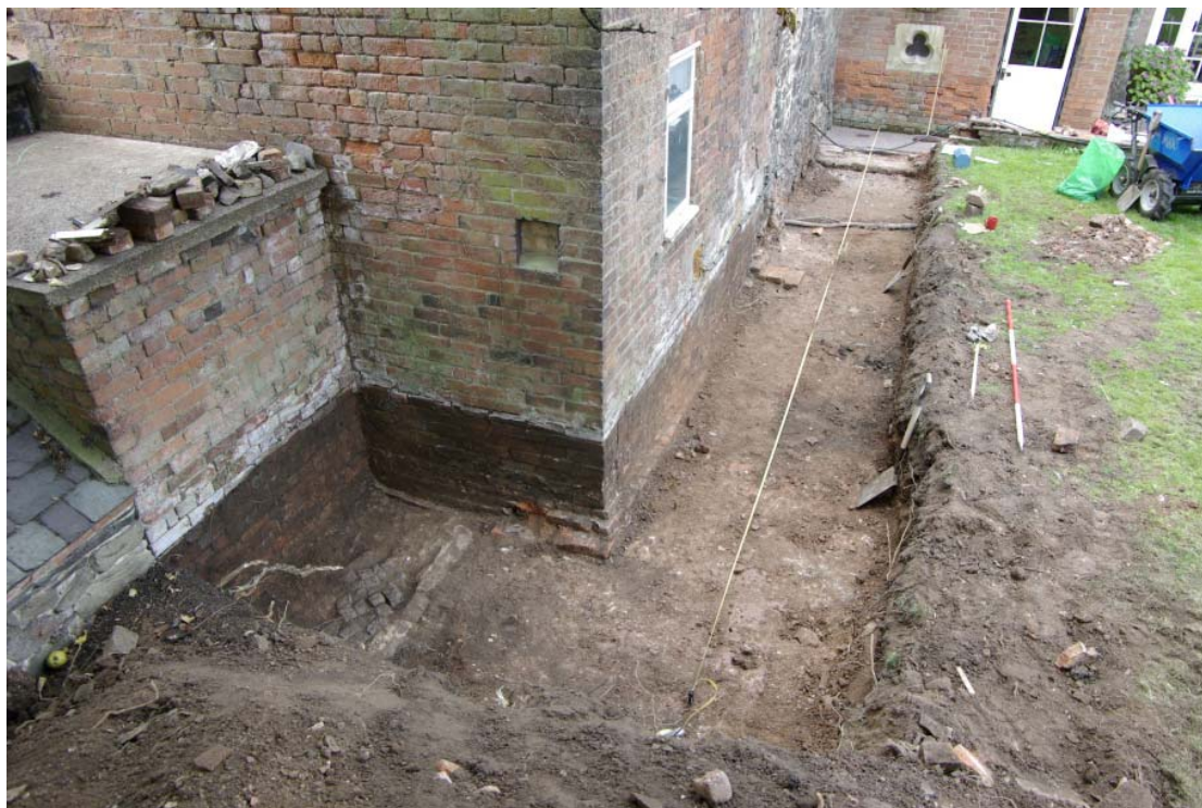
Photo 1. The excavated trench, looking south.
