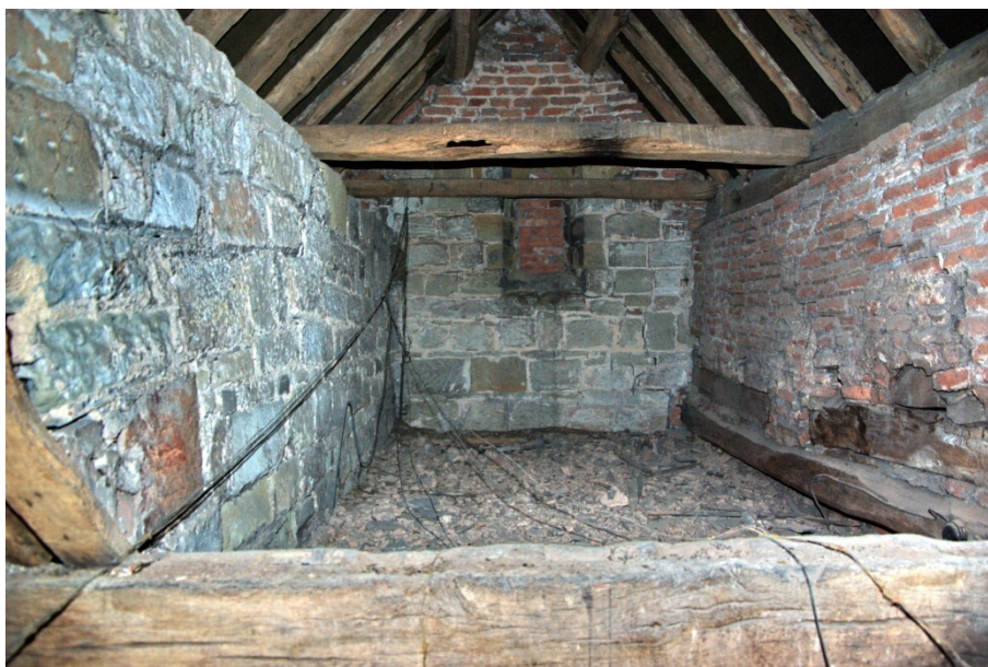
Photo. 9. Former attic room Range F, reused stonework and blocked window
