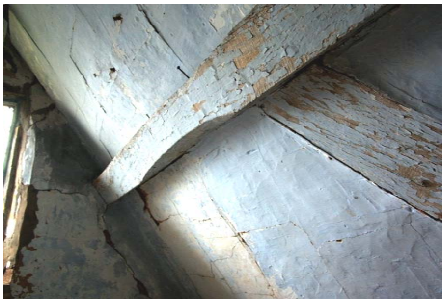
Photo. 10. Trimmed purlin in Range G indicating former door into adjacent attic room
