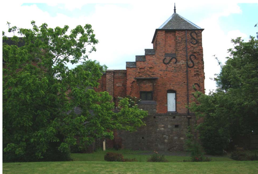
Photo. 4. Tower B from the NW showing 1 st & 2 nd floor doors and splayed window opening to 'lost' Range D
