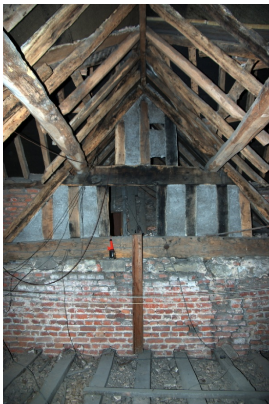
Photo. 1. Smoke-blackened 15 th century roof truss over former open hall (Range A)
