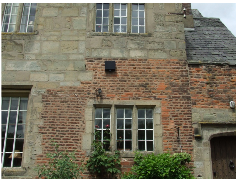
Photo. 8. Early brickwork in the lower section of Range F
