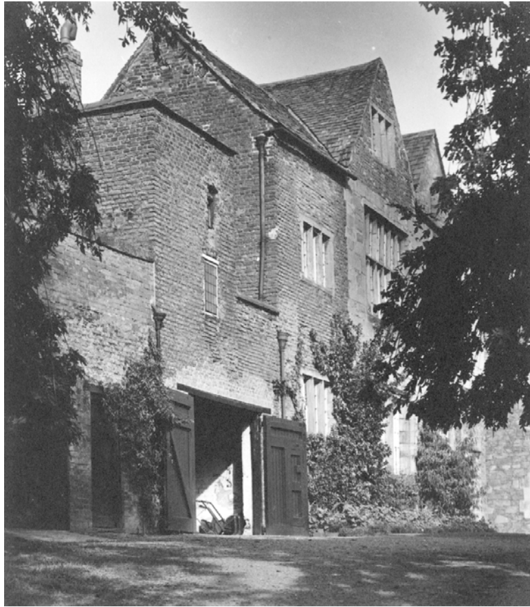
Figure 27. Groby Old Hall from the south showing garage enlarged between 1912 & 1923.
