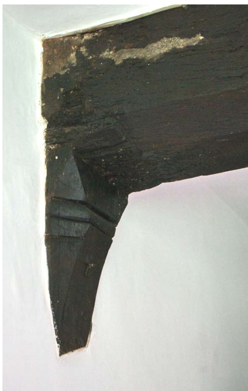
Photo. 2. Moulded bracket supporting inserted floor in former open hall
