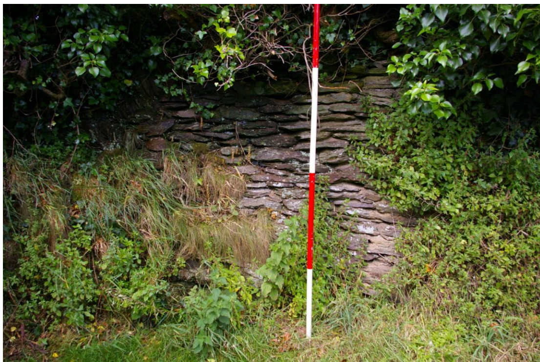
Figure 19: 75634, External wall of small building from east.
