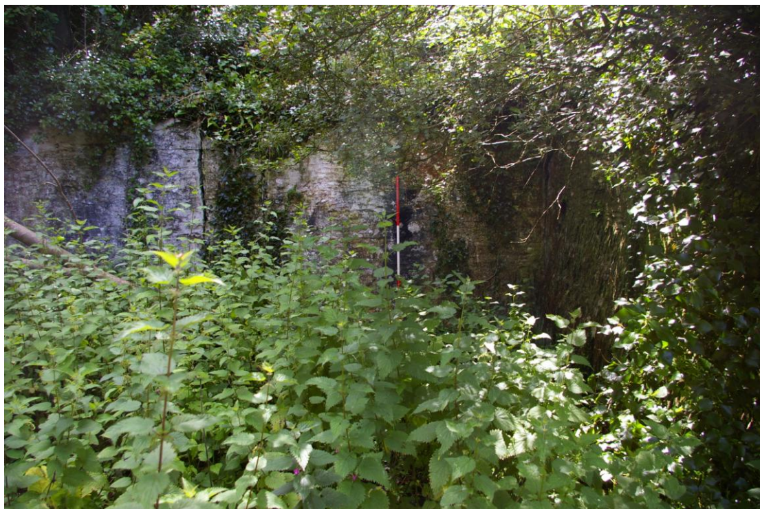
Figure 17: 75630: Interior of roofless shelter from north
