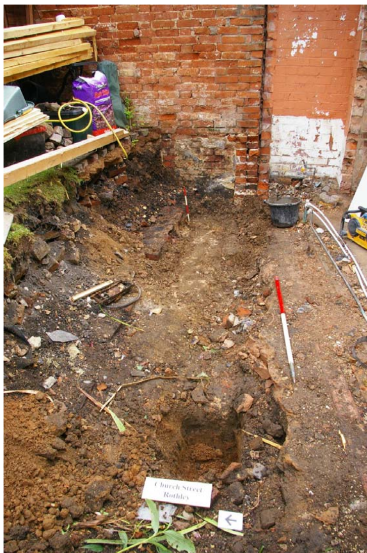
Figure 5 Existing footings & trial hole in foreground (looking east).
