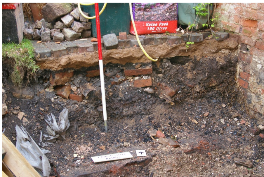
Figure 4 Made ground exposed behind retaining wall (looking north).
