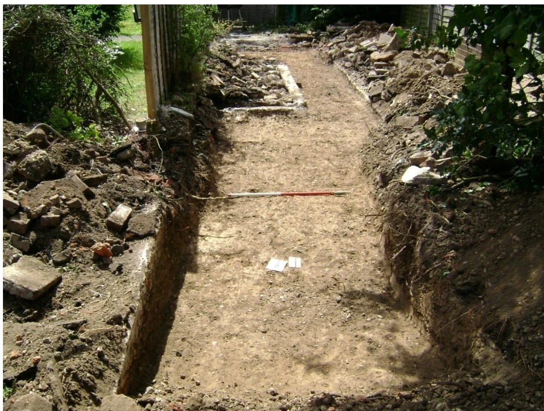
Figure 8. Trench after initial 10 metre excavation Looking south-east, 1m scale.
