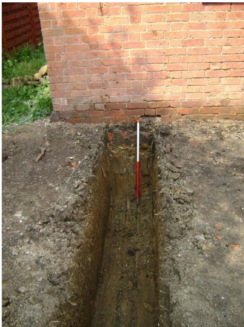
Figure 8 Foundation trench at joint with existing barn Looking north. 1m scale
