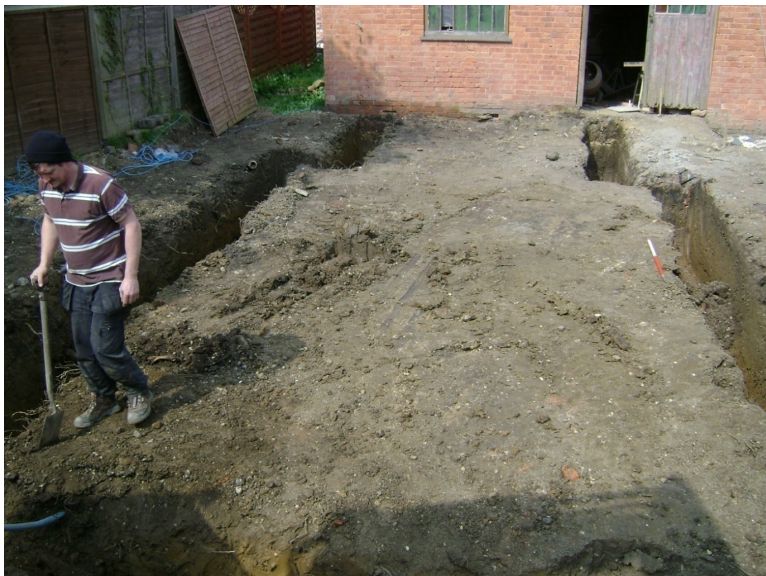
Figure 6 Excavated foundation trenches Looking north. 1m scale
