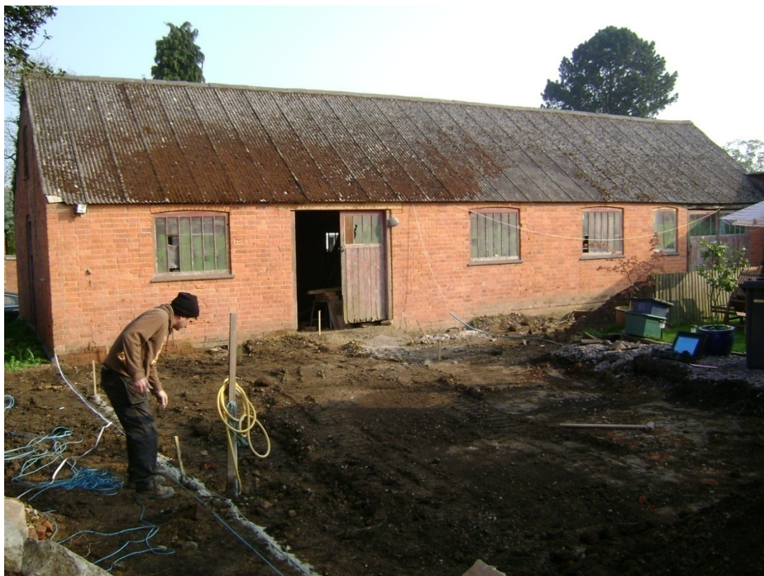
Figure 4 Location of extension prior to excavation of foundations Looking north-east
