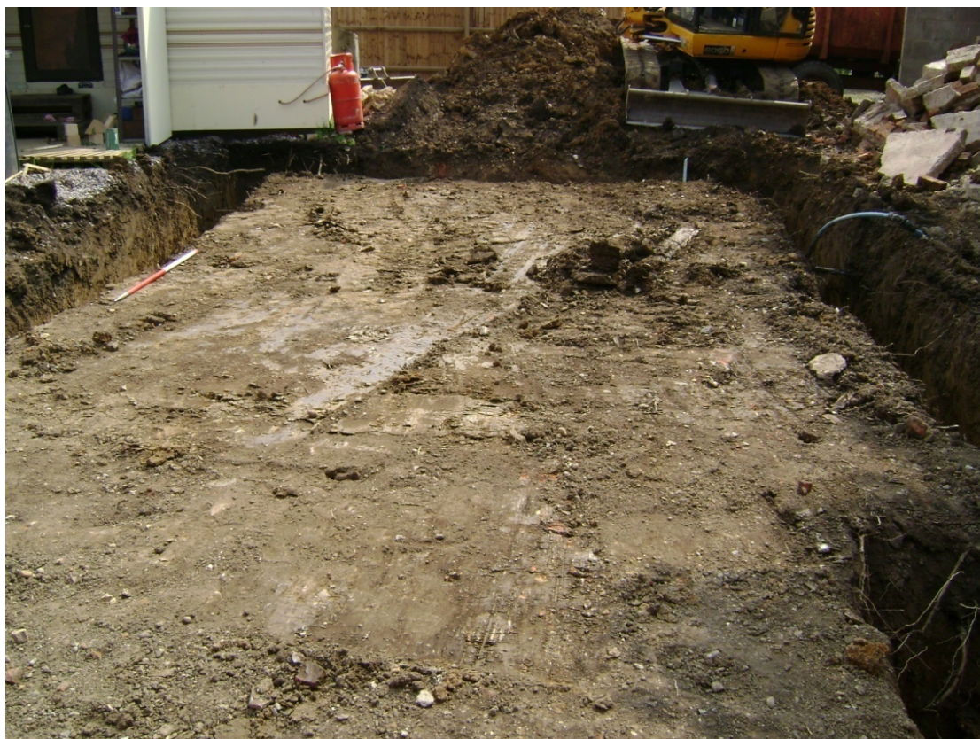
Figure 7 Excavated foundation trenches Looking south-east. 1m scale
