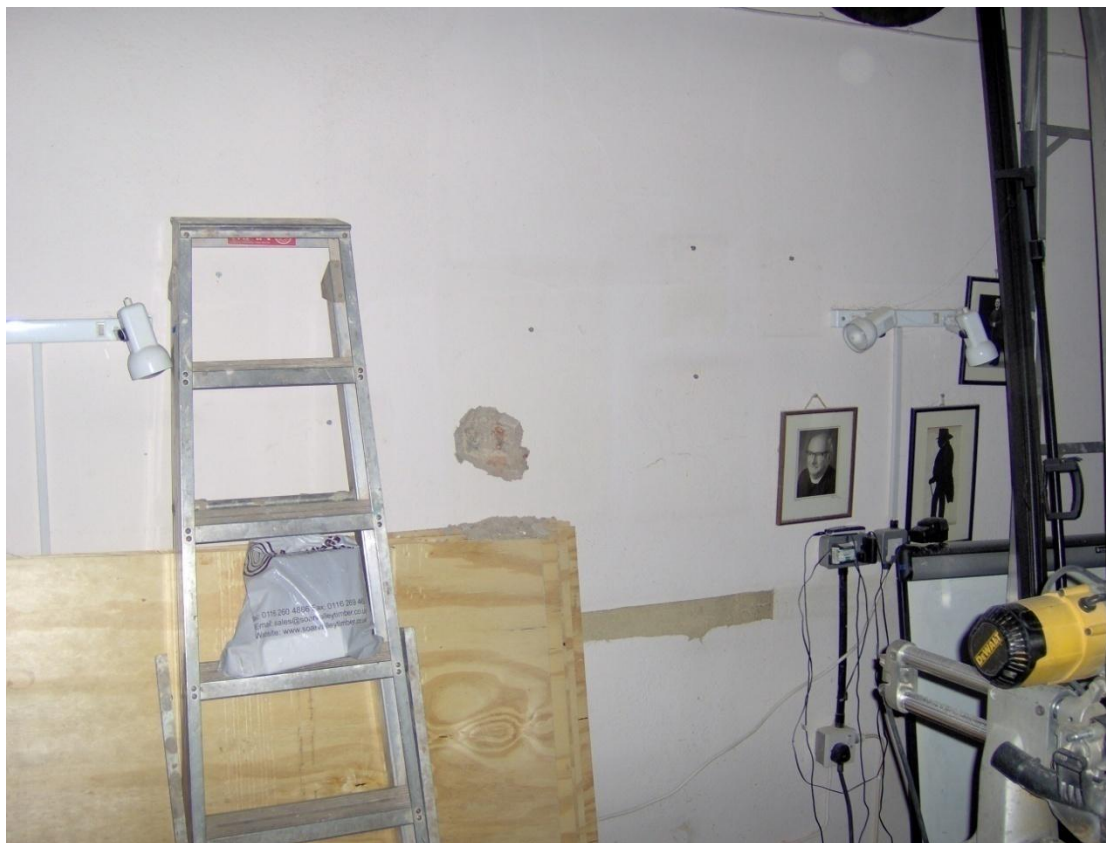
Plate 6: Area of work in north transept showing test-slot, looking west
