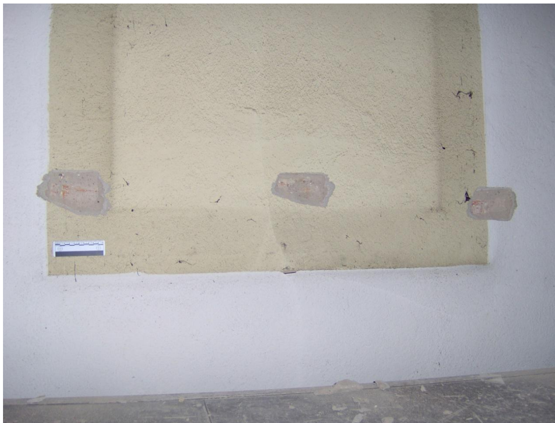
Plate 4: Test slots showing brickwork in the north aisle, looking north
