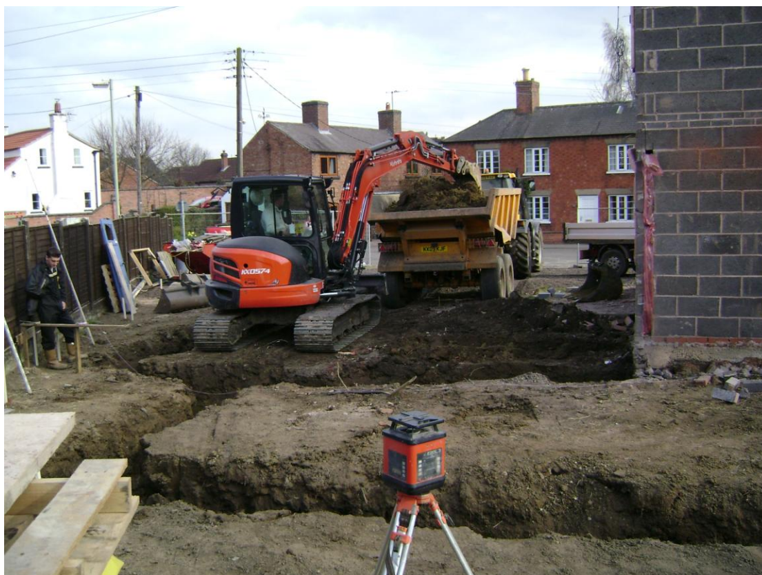
Figure 8 Foundation trenches on north-east side of house looking east
