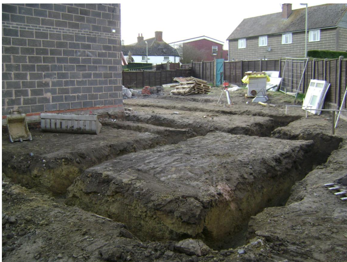
Figure 9 Final foundation trenches looking south-west
