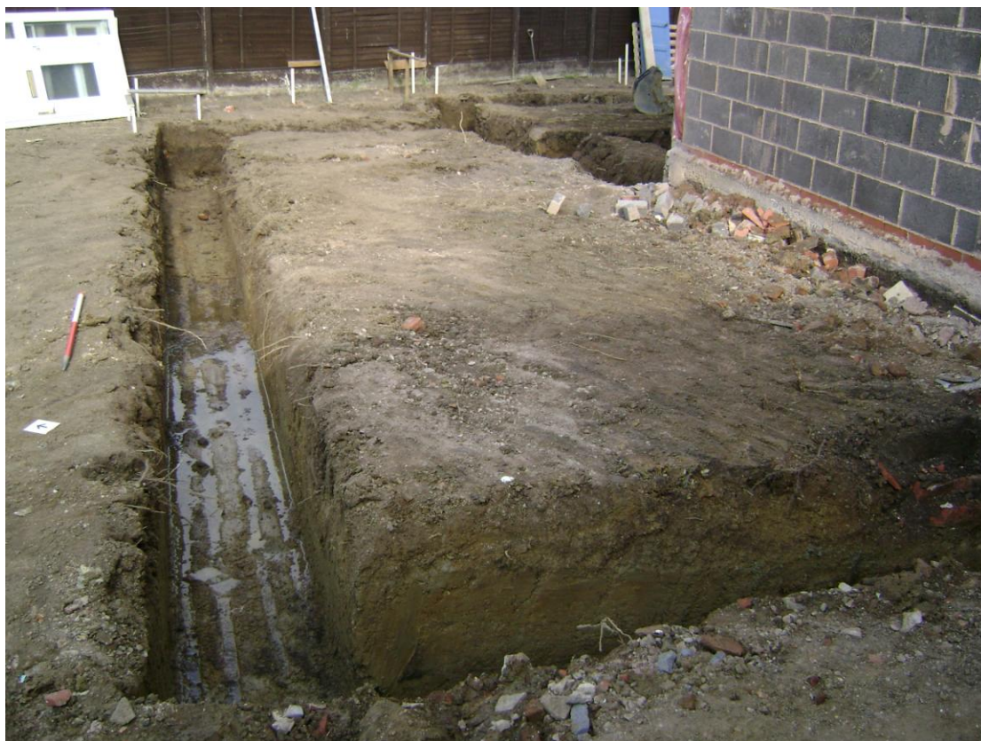
Figure 7 Foundation trenches on north-west side of house Looking north-east. 1m scale
