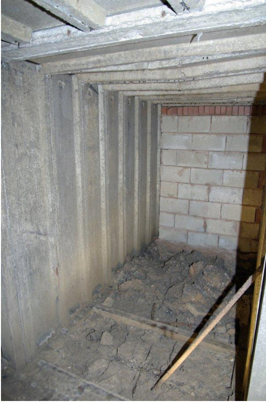
Figure 12 Southernmost blocked trench.
