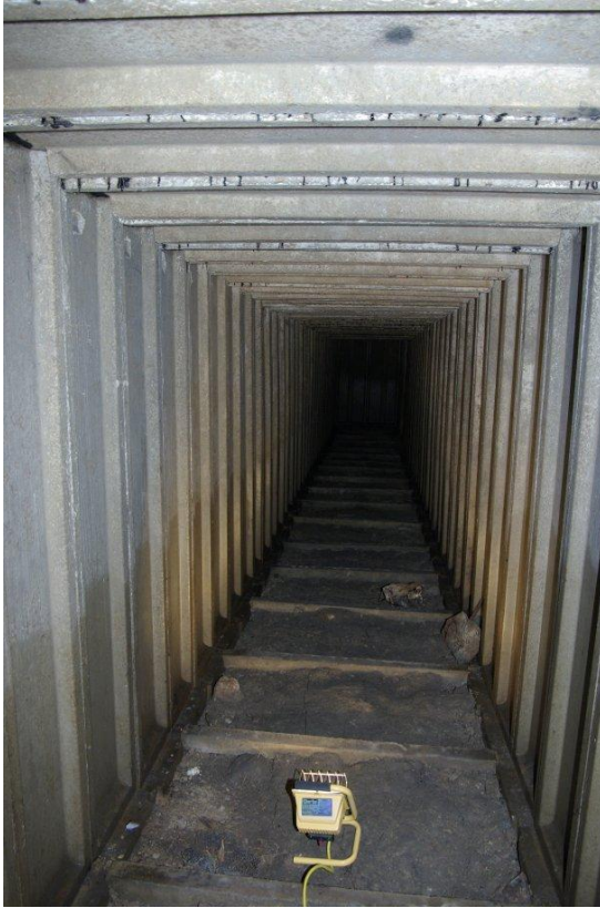
Figure 10 Northernmost trench (looking east).
