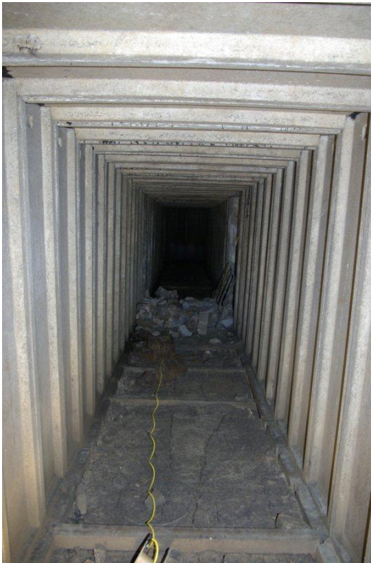
Figure 8 Southernmost trench (looking east).
