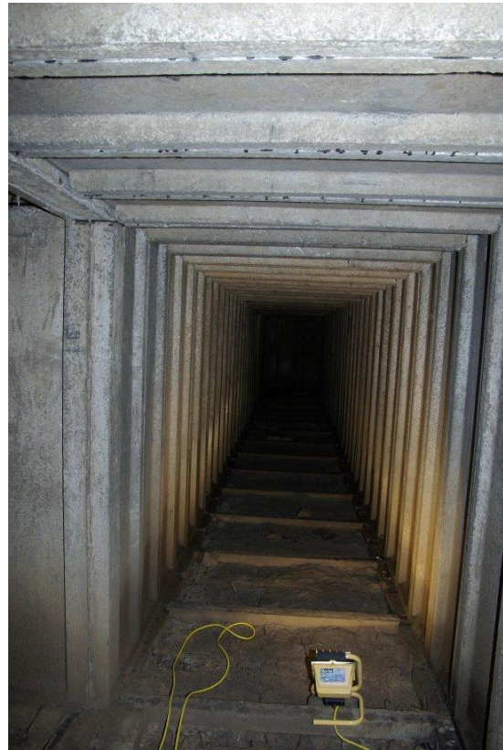
Figure 9 Westernmost trench (looking north).
