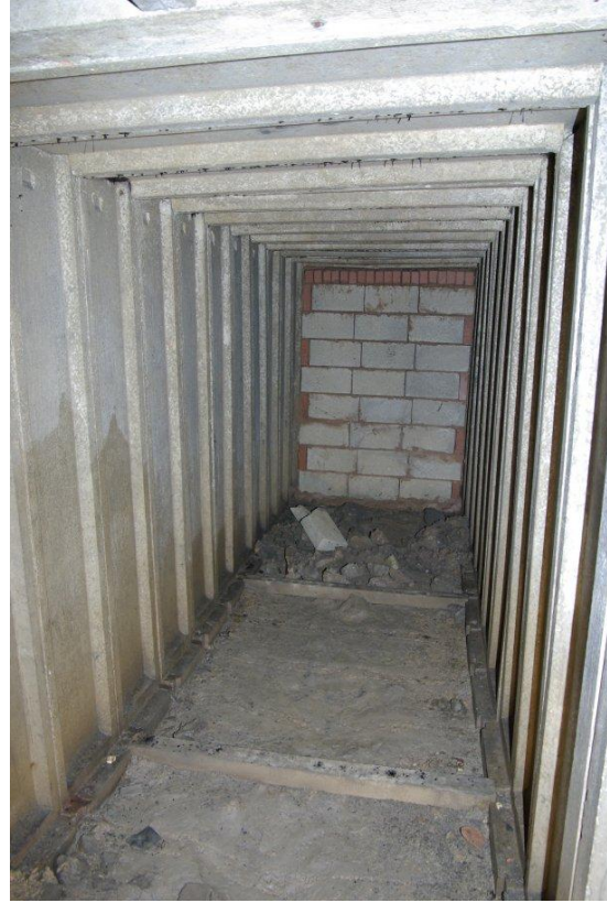
Figure 13 Northernmost blocked trench.
