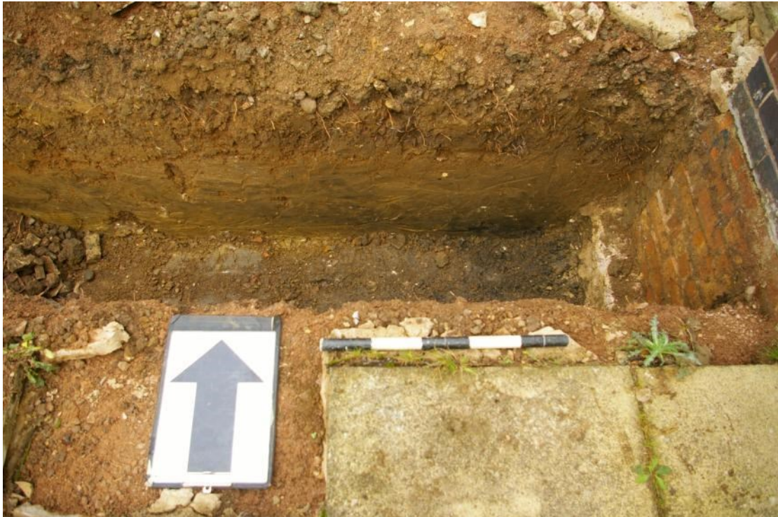
Figure 4: Section through overburden and subsoil for rear extension trench 1. Photographic scale 0.5m
