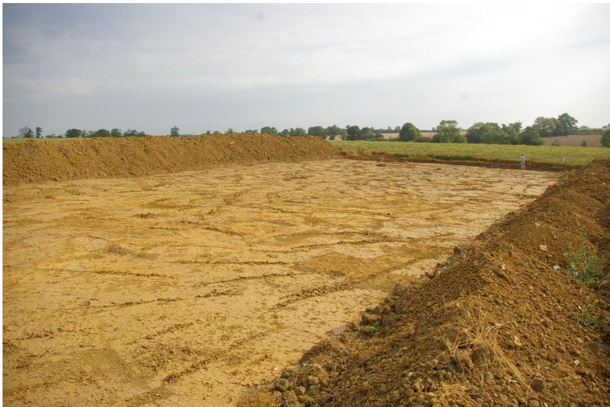
Figure 18: Turbine 11 during excavation, looking north-east
