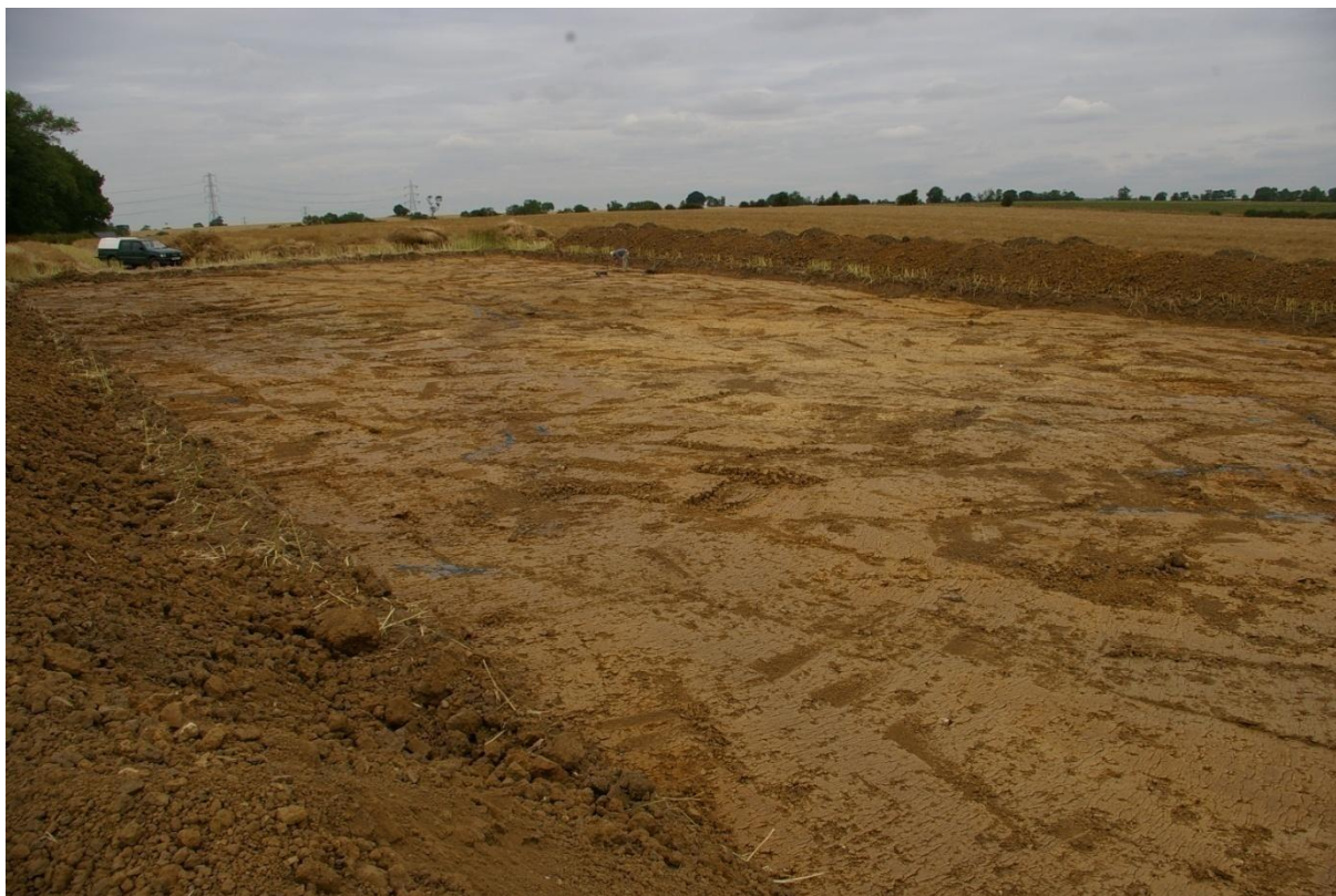
Figure 17: Turbine 9 during excavation, looking north
