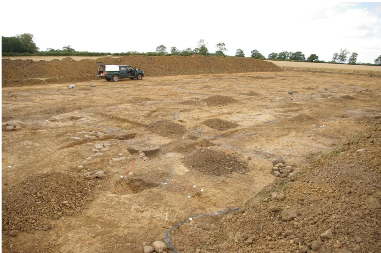
Figure 3: Turbine 4 during excavation, looking north-west
