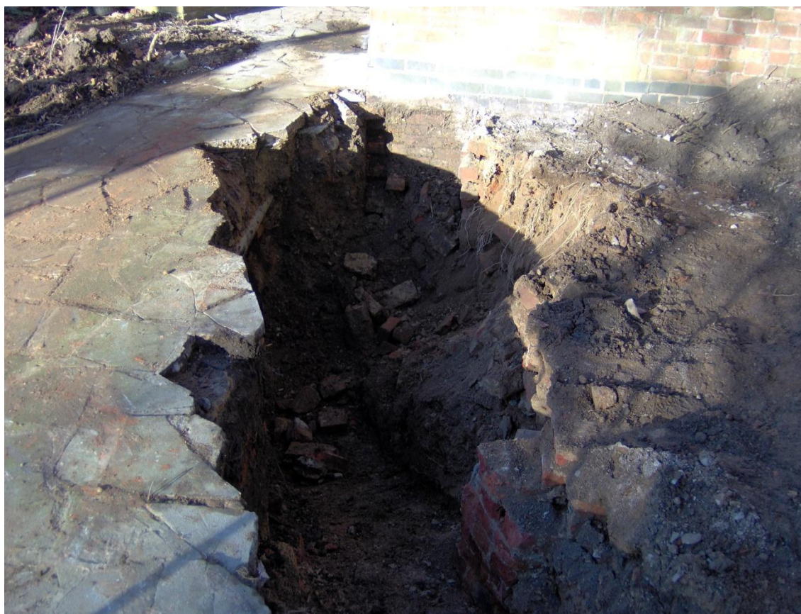
Figure 4: Photograph showing brick footings and the brick-filled void of a former extension of the farm house, looking north
