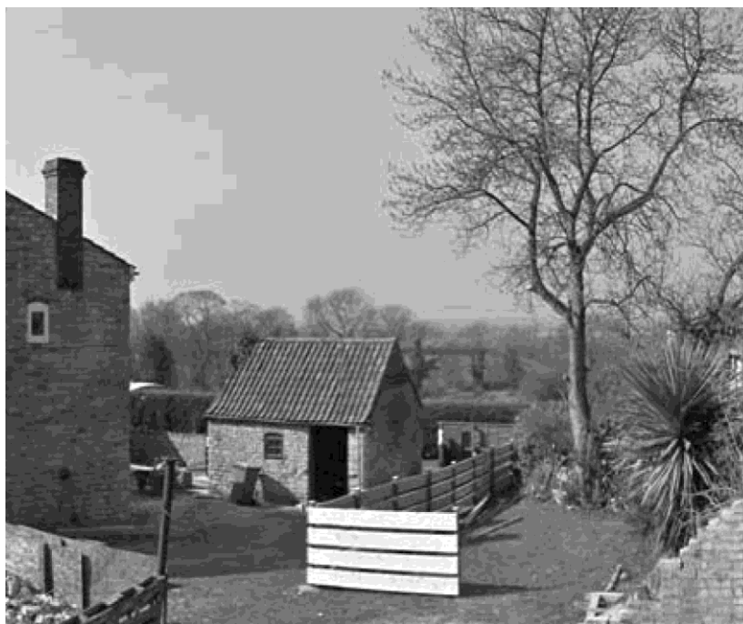
Figure 4. Single storey structure demolished to make way for new garage. Looking south-west.
