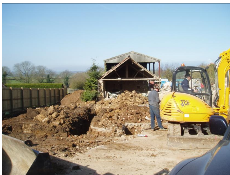
Figure 18. Excavation of footings for house plots 1a and 1b. Looking west.
