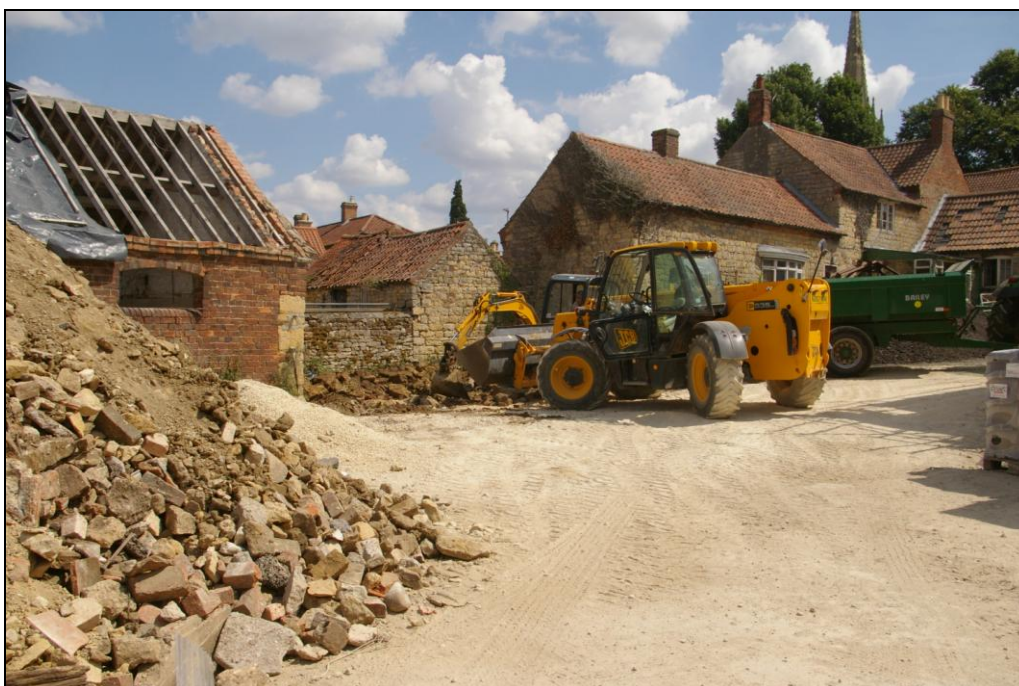
Figure 27. Excavation of footings on eastern side of 19th century cowshed.
