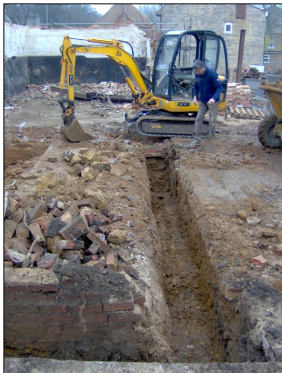
Figure 14. Footings for new single garage, looking south along western trench.
