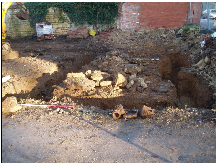
Figure 12. Footings for double garage, looking north.
