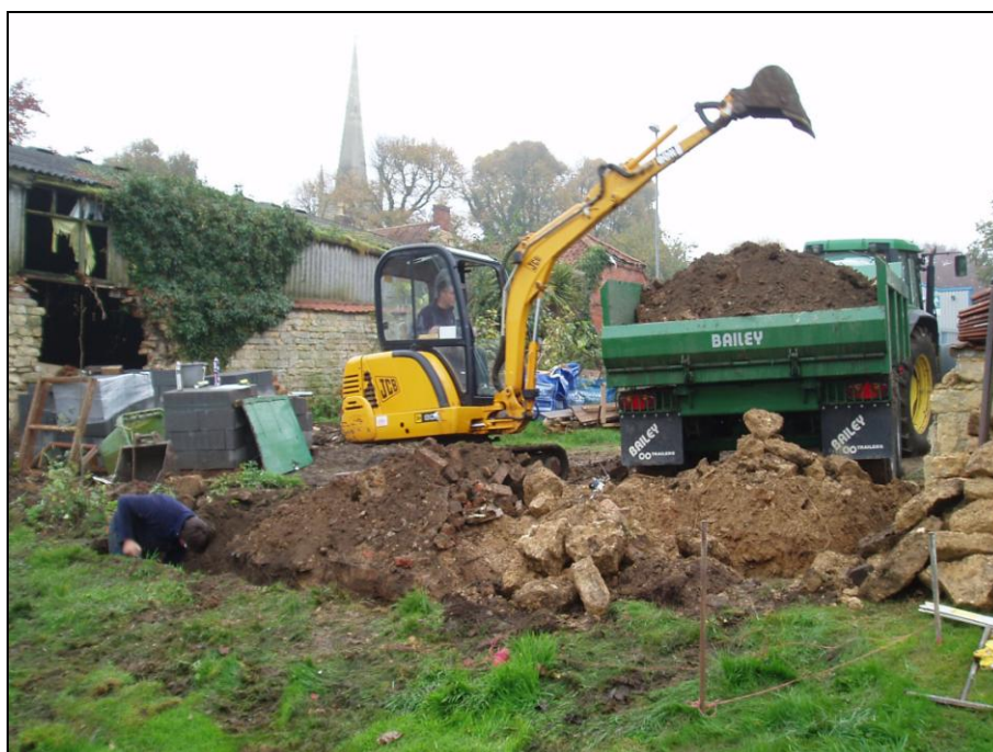
Figure 8. Footprint of new garage, looking east.
