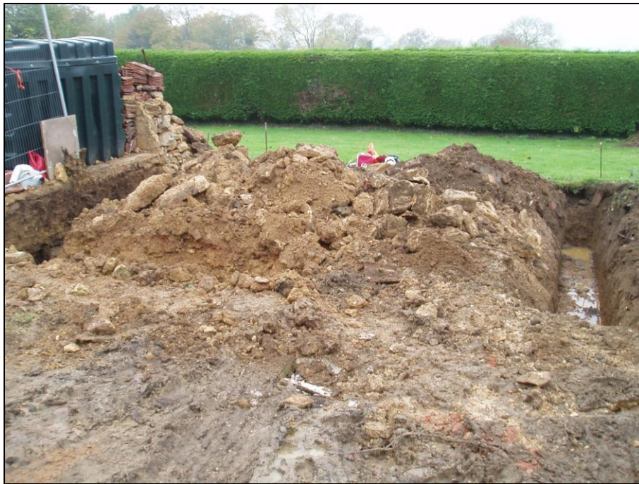
Figure 7. Footprint of new garage, looking west.
