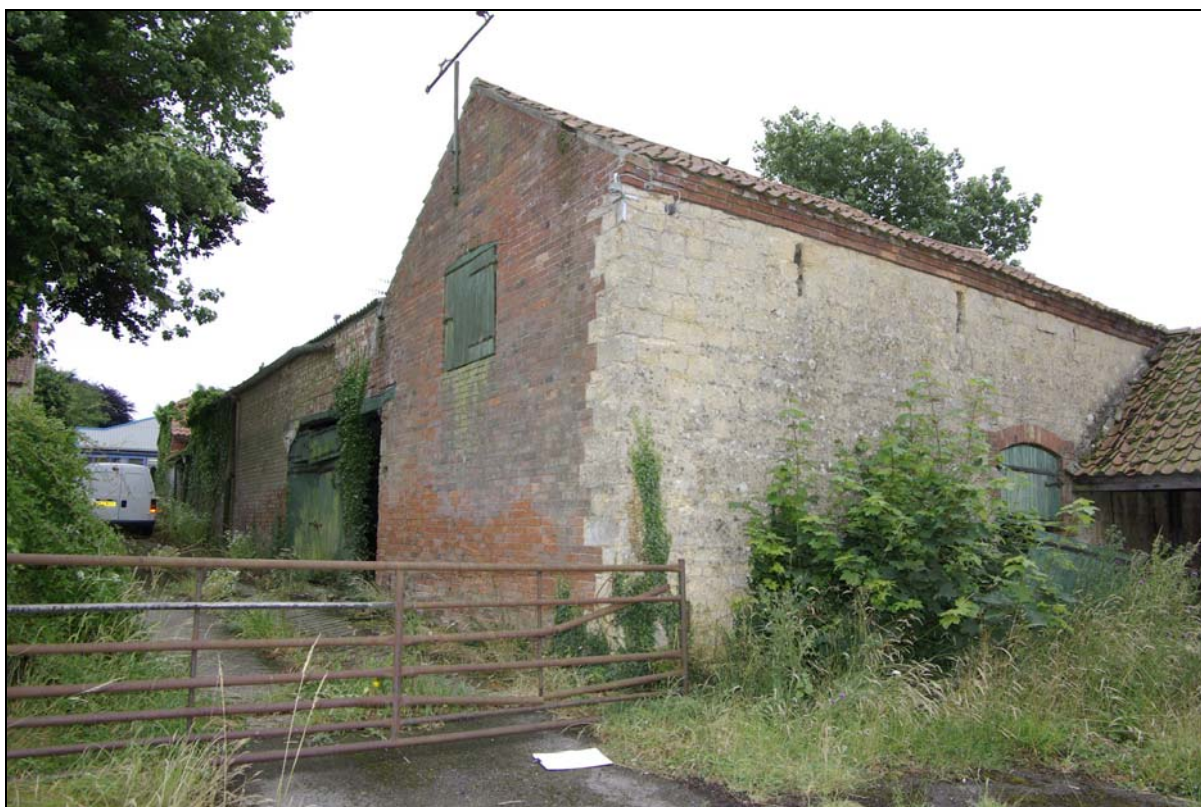
Plate 22. Stone and brick-built barn. Looking south east.
