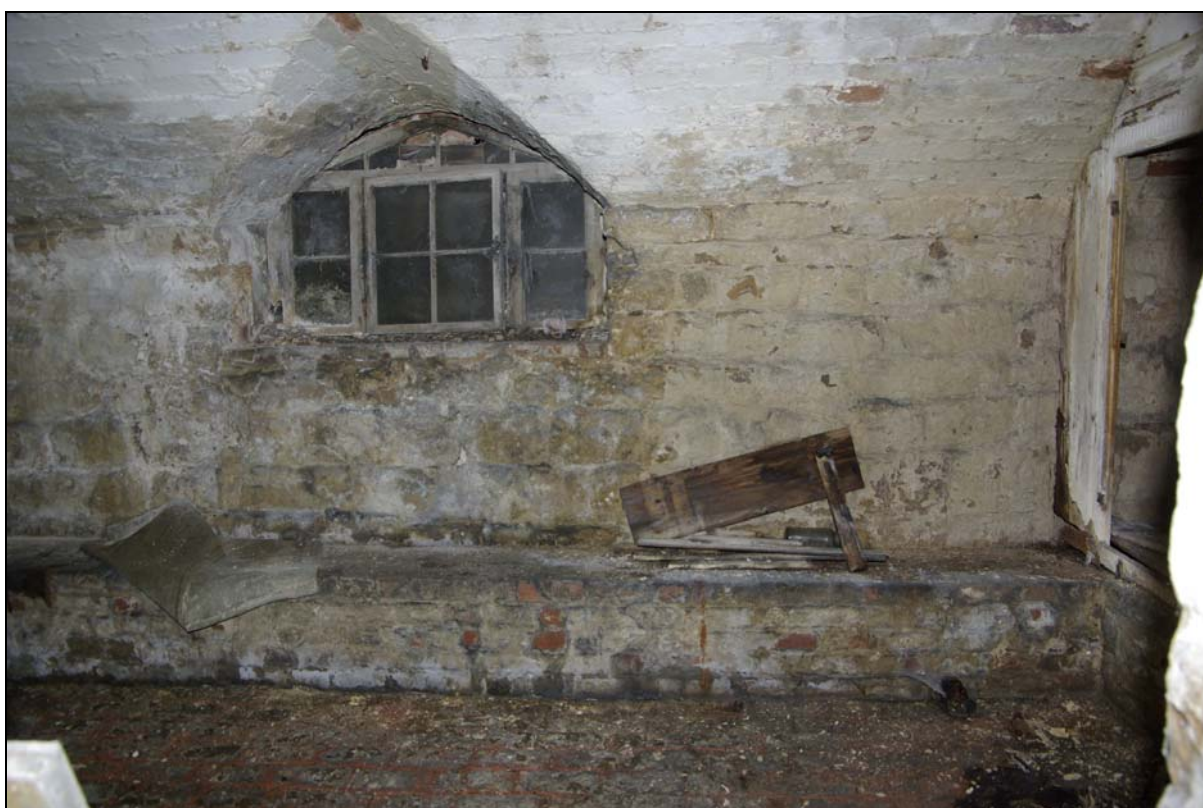
Plate 11. Stone cellar, with vaulted brick ceiling and thrall. Looking south.
