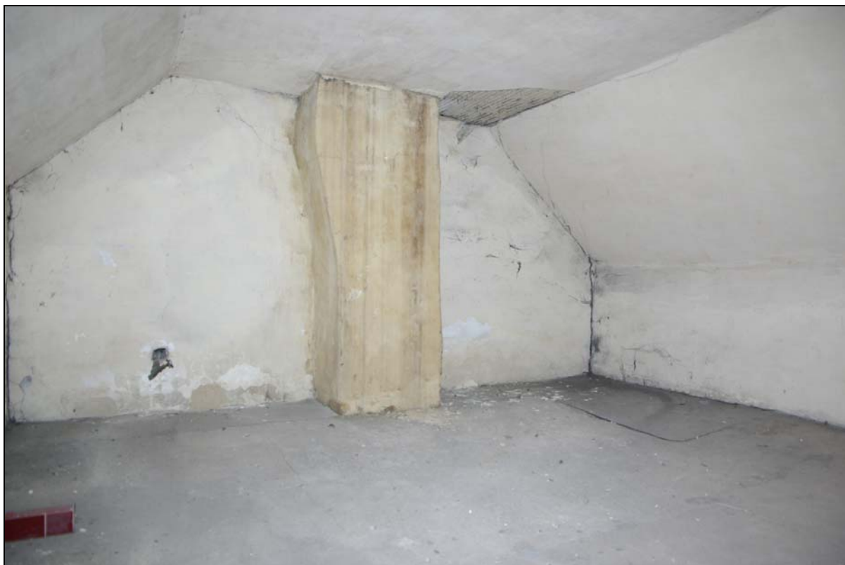
Plate 16. First floor store-room with lime ash floor. Looking north.
