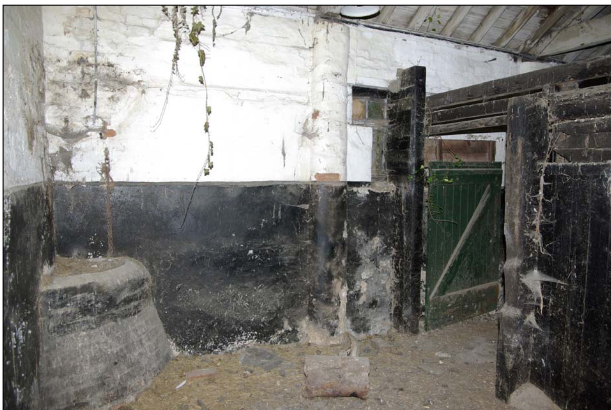
Plate 31. Brick trough in stable (cast iron hayrack removed). Looking west.
