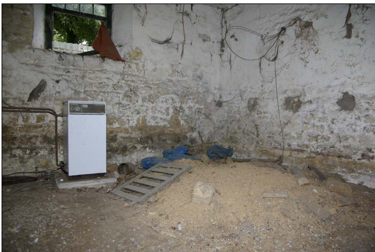
Plate 19. Former workshop and woodstore, with modern boiler. Looking south-west.
