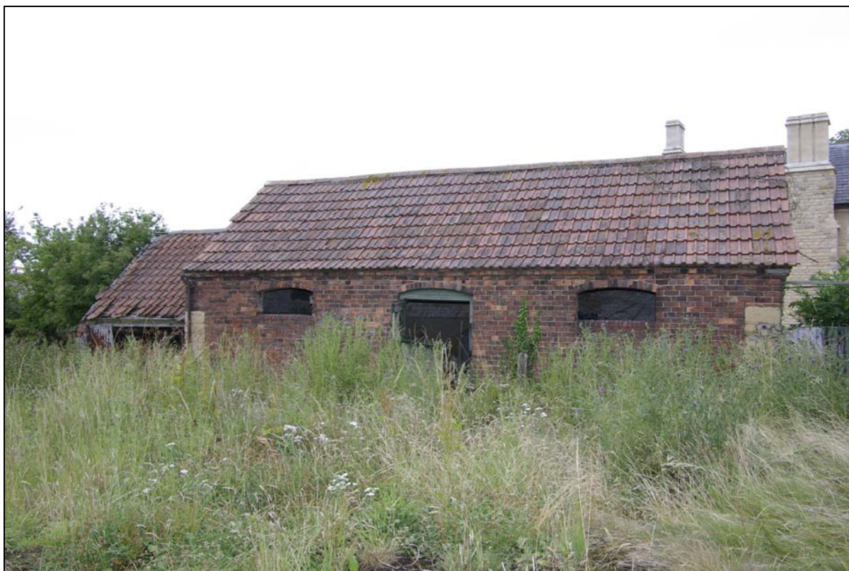
Plate 34. Brick cow-shed, located on western side of farmstead. Looking north.
