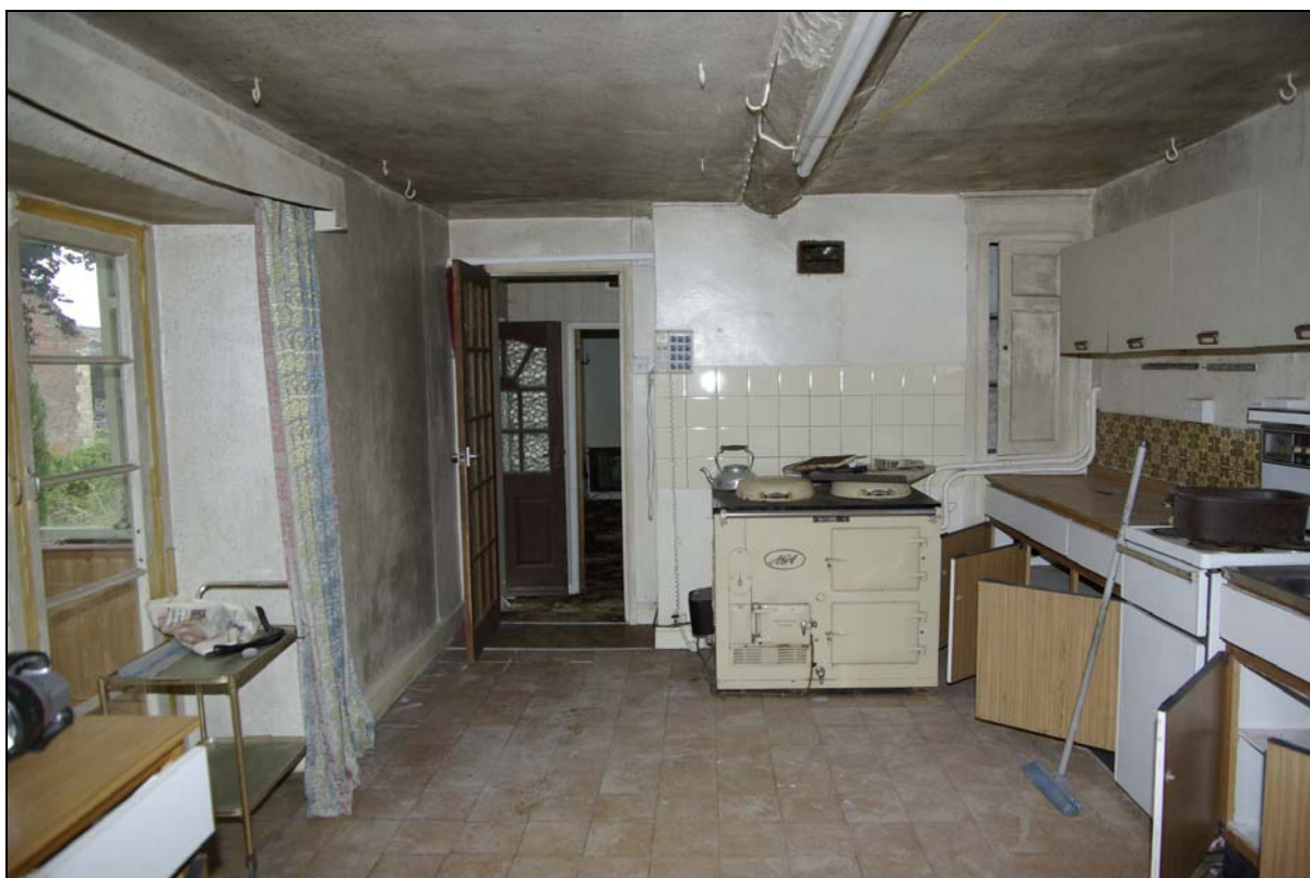
Plate 7. Kitchen, with chimney stack and early built in cupboard. Looking south
