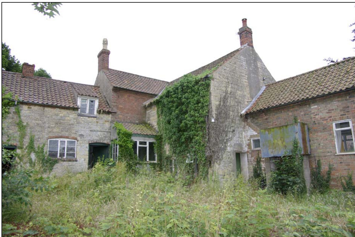
Plate 3. As above, looking south-east.
