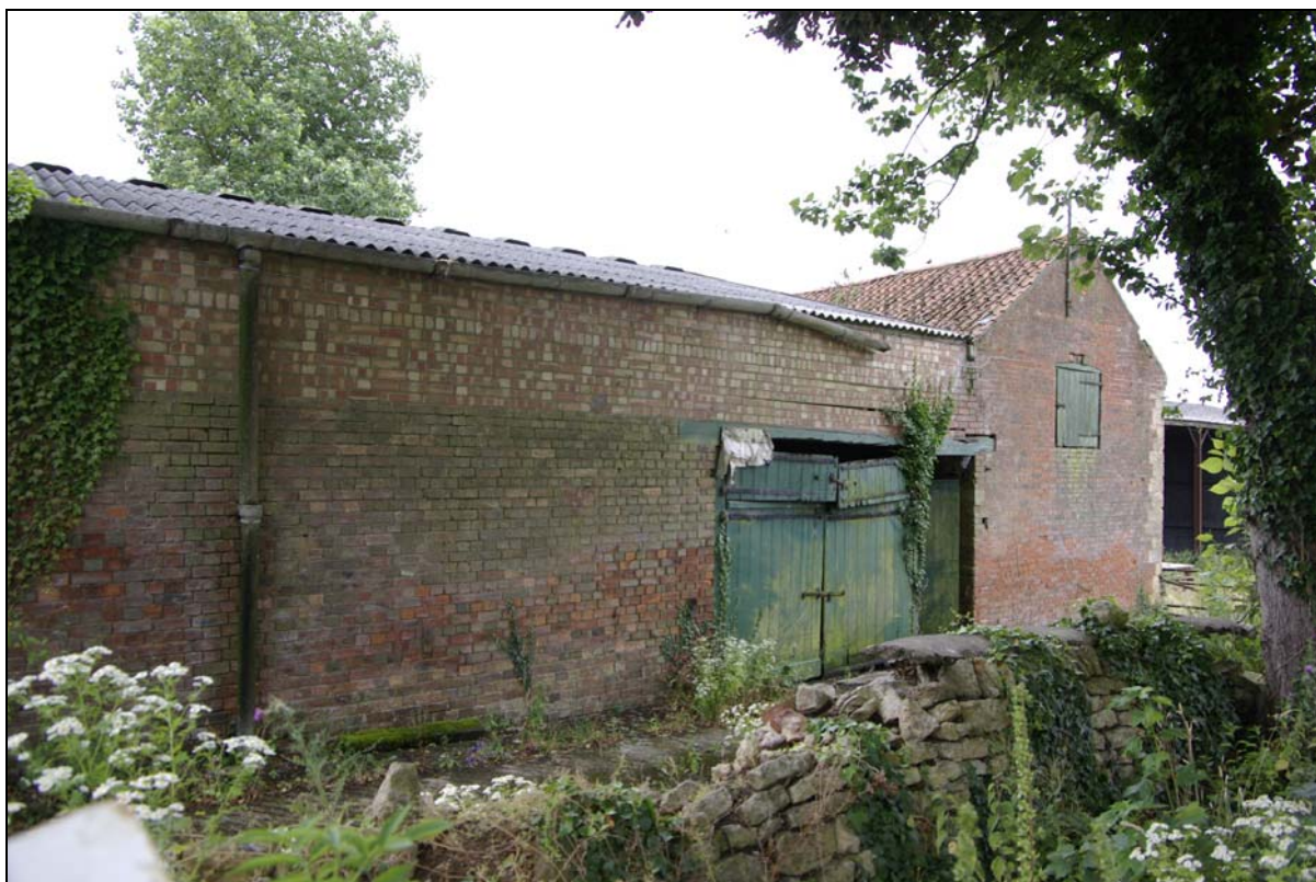
Plate 21. Infill structure between cow-shed and barn. Looking west.
