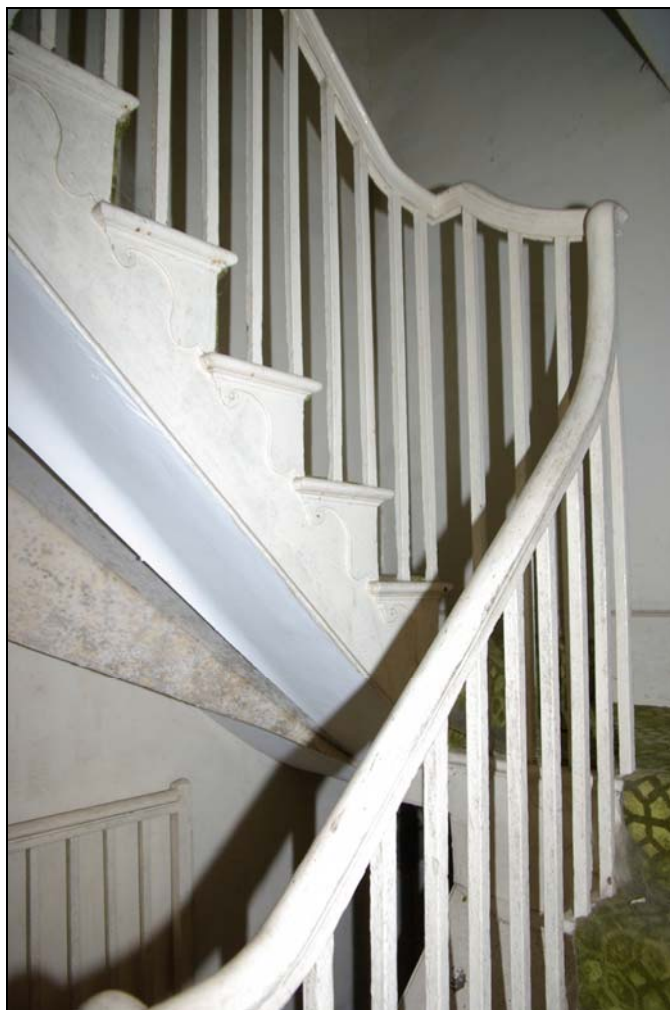
Plate 9. Open-string staircase, with moulded handrail and decorative brackets. Looking west.
