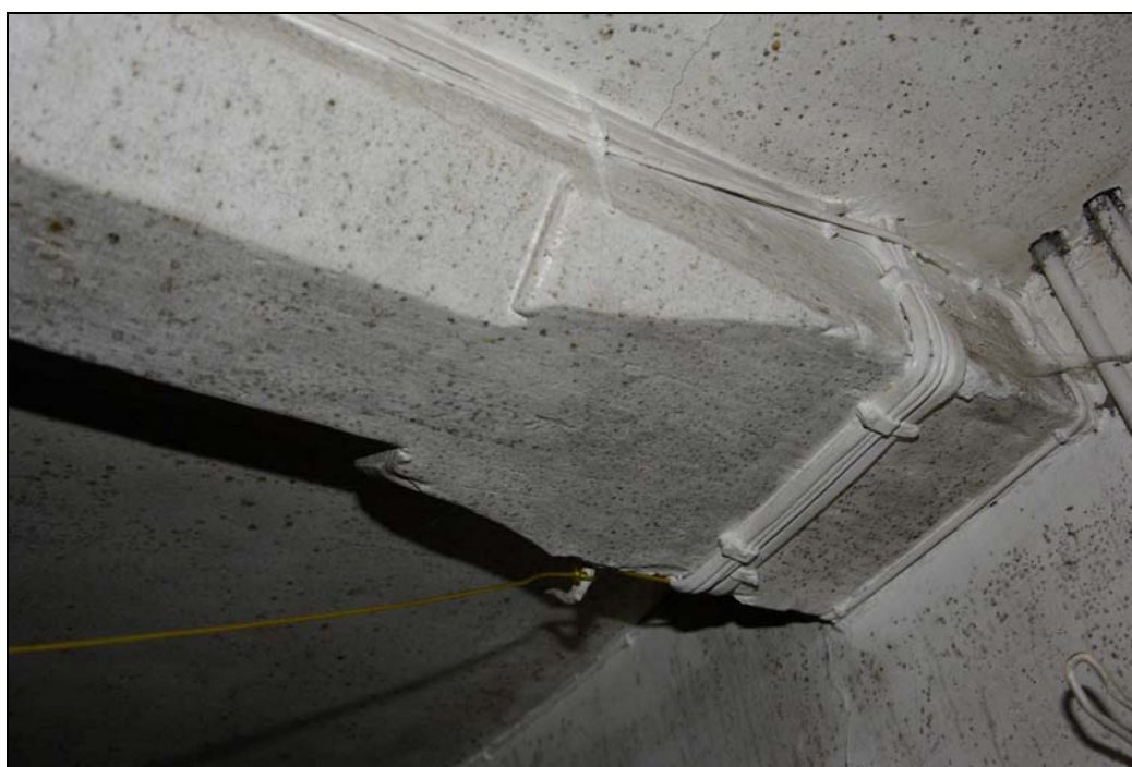
Plate 8. Chamfered and stopped axial beam in kitchen. Looking north-east.
