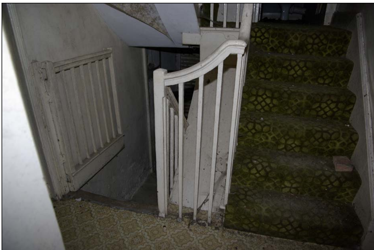
Plate 10. Dog-gate, opening onto cellar steps. Looking west.
