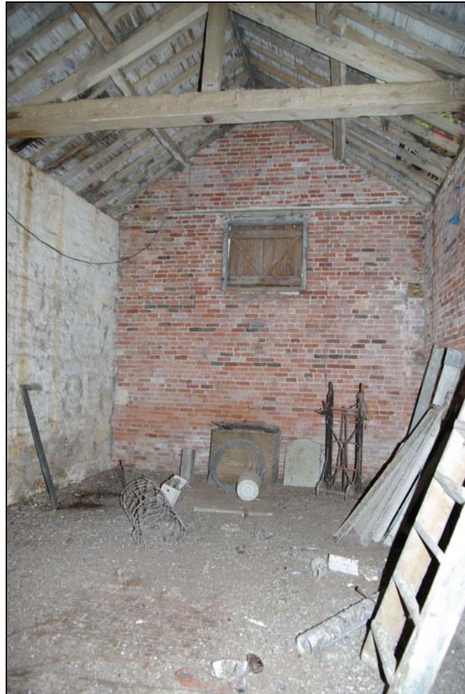
Plate 26. Barn interior. Looking north.
