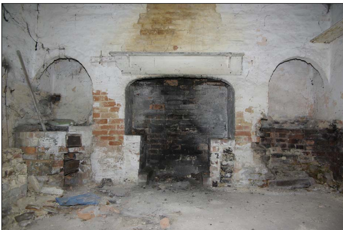
Plate 17. Washhouse, with hob-grate fireplace and cast-iron 'coppers' removed. Looking north.
