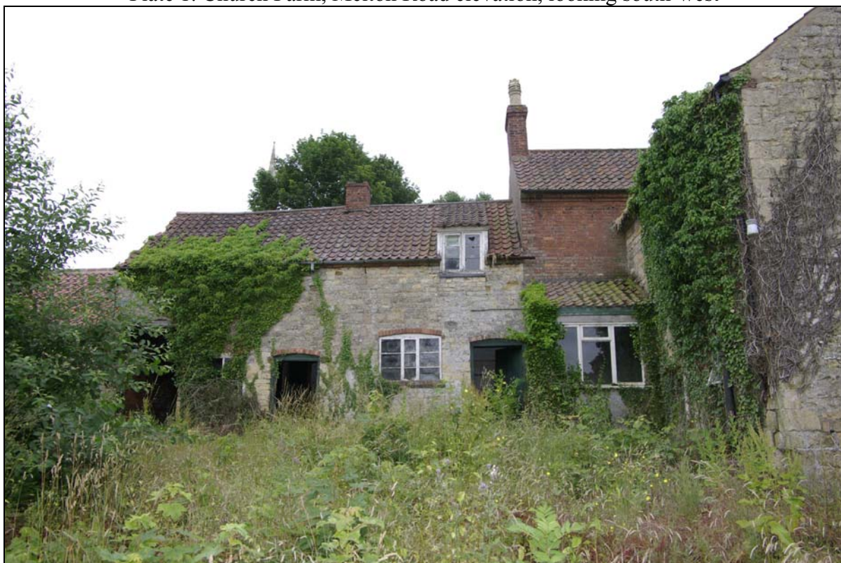
Plate 2. Farmyard elevation, looking east
