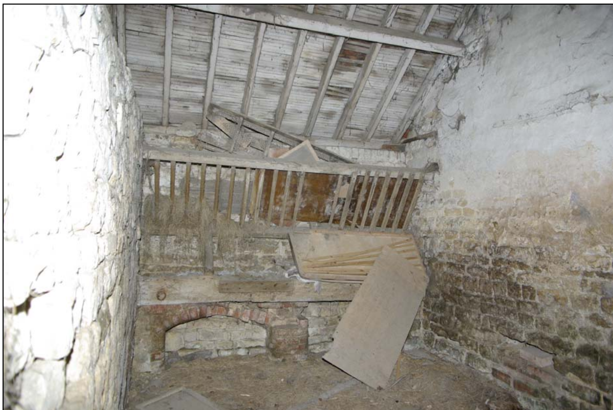
Plate 33. Stable interior, with timber hayrack. Looking west.
