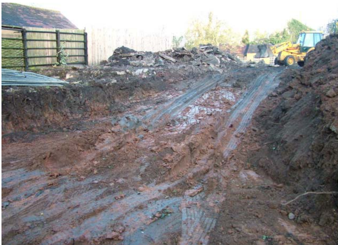
Plate 4: Entranceway after excavation but before laying hardcore
