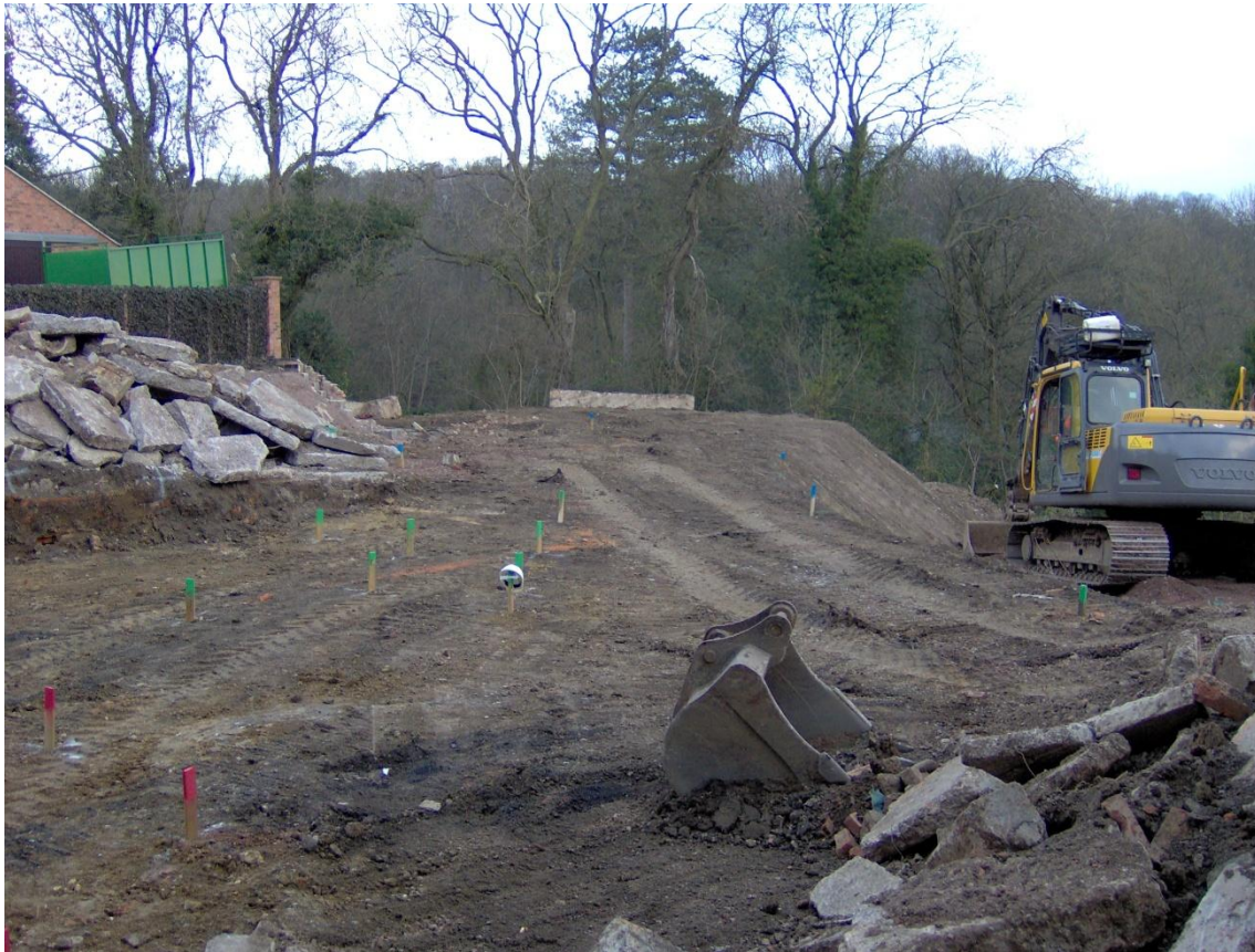
Figure 3: The project area before evaluation, looking north
