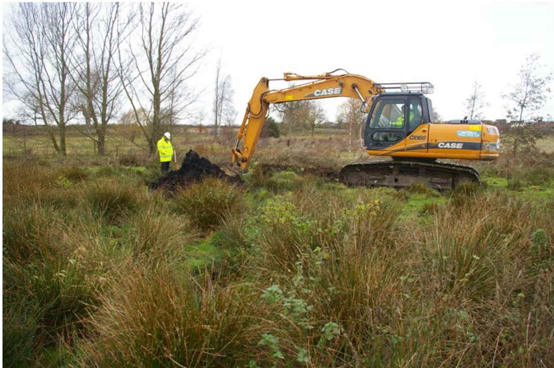
Plate 4: Work in progress within marshy area, Trench 6, Field 1, looking west
