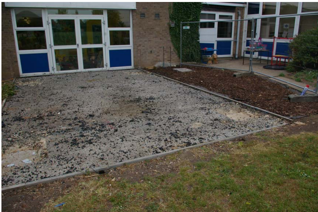
Plate 1: Site cleared prior to excavation, looking north
