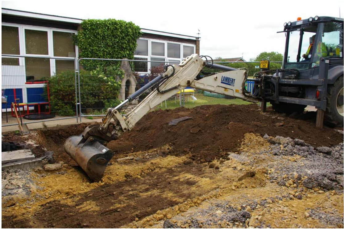
Plate 2: Work in progress, looking east
