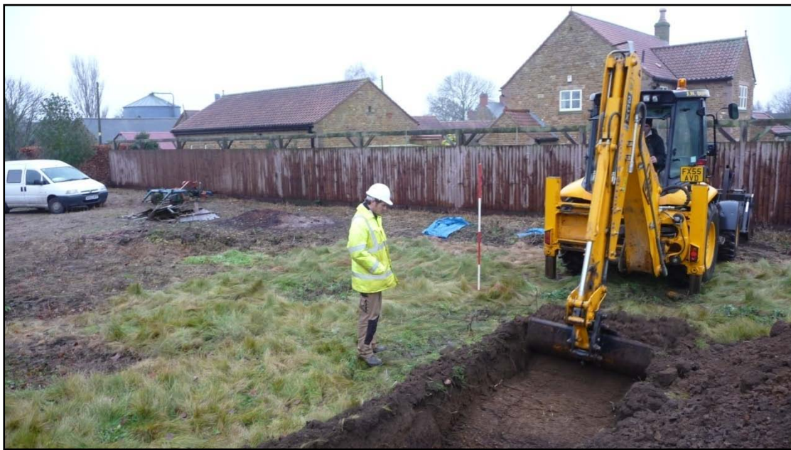
Figure 3: Machining of Trench 1 in progress; view south-east
