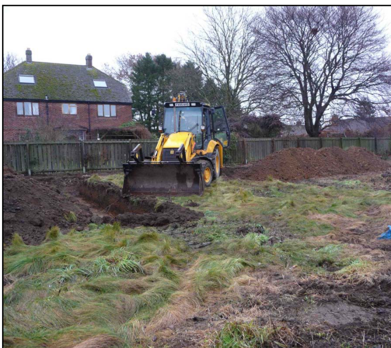
Figure 5: Trenches 1 & 2; general view north-east
