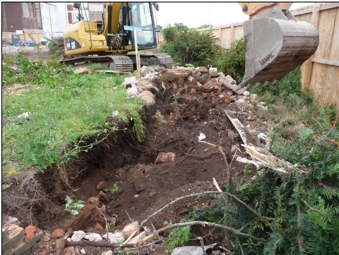
Figure 9: Machine removal of western retaining wall; view west
