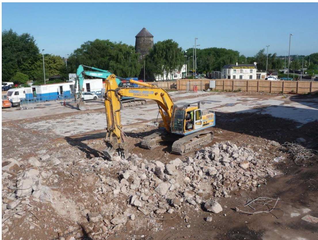
Figure 4: Northern building floor slab breaking in progress; view northwest
