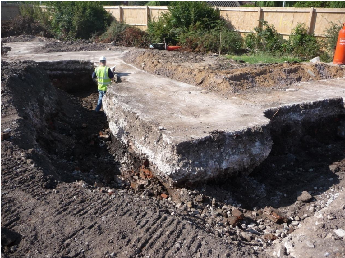
Figure 8: Western ring beam foundation exposed; view south-west
