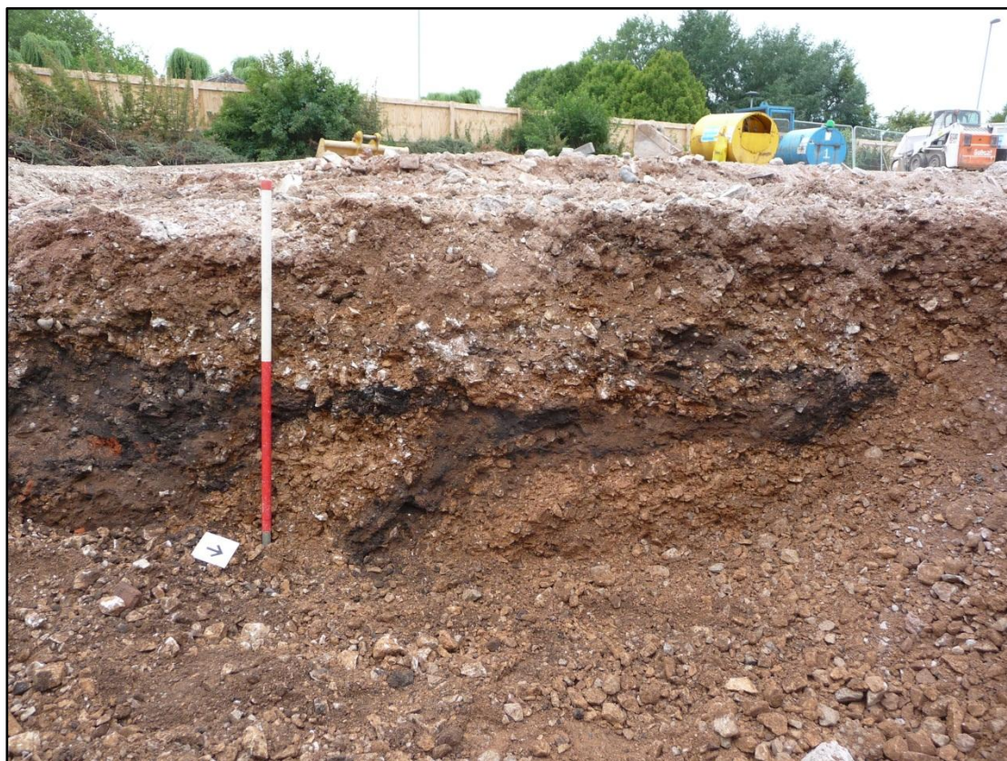
Figure 6: Vibro-compacted roadstone revealed in section flowing removal of foundation pad. View west; 1m scale
