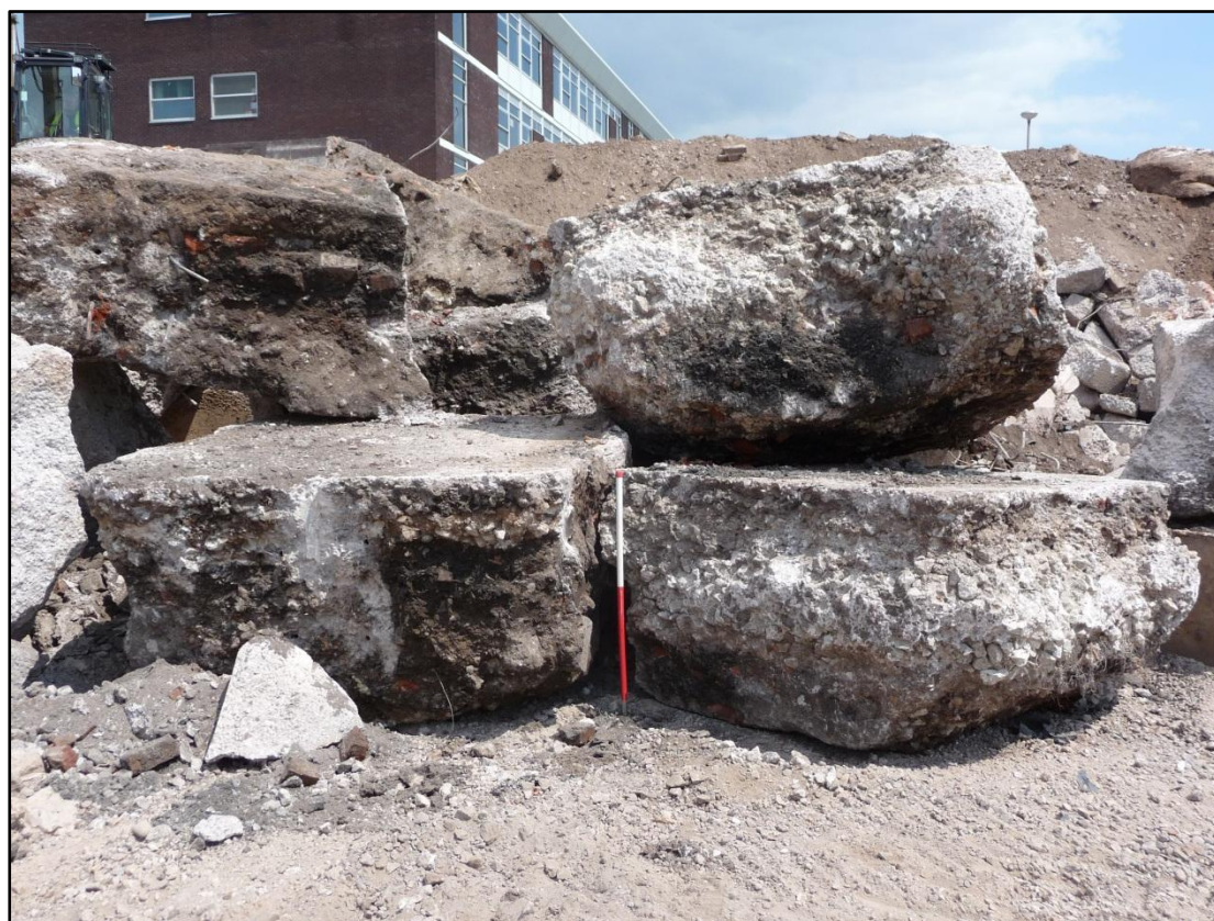
Figure 5: Concrete foundation pads; 1m scale
