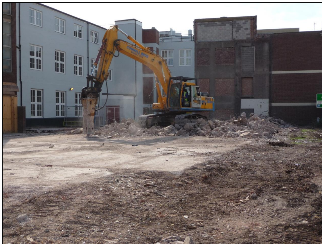
Figure 15: Breaking of southern floor slab in progress; view looking south-east
