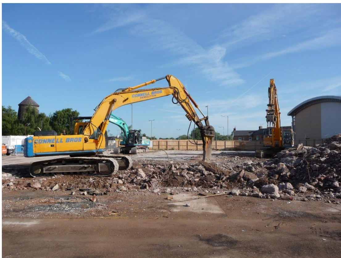
Figure 3: Northern building floor slab breaking in progress; view northwest
