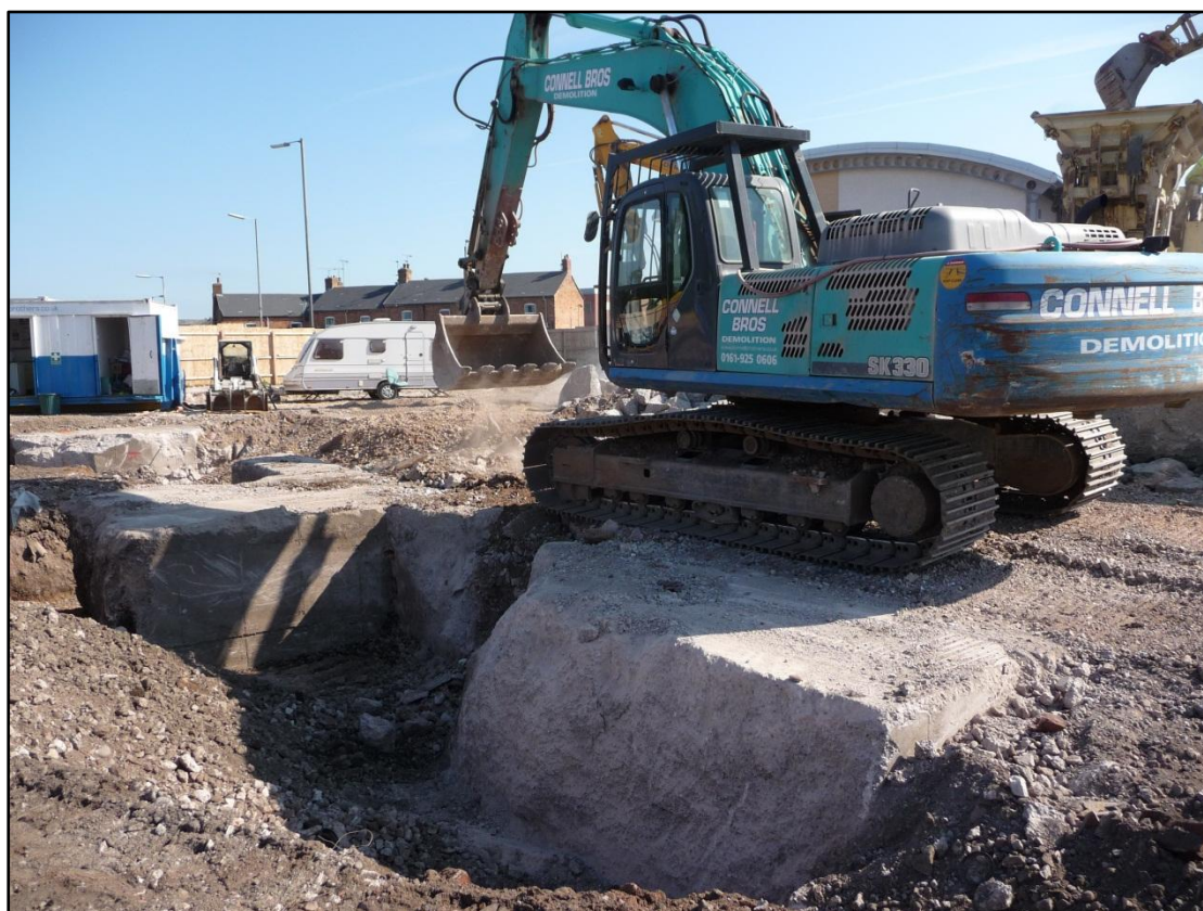
Figure 7: Removal of foundation ring beam in progress; view north
