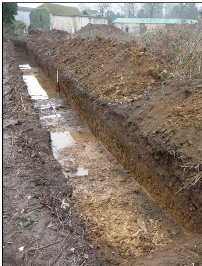
Figure 5: Trench 1: view south-east; 2m scales
