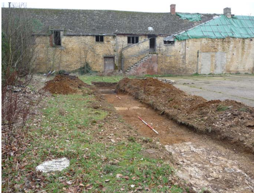
Figure 21: Trench 3: general view north (2m scales)
