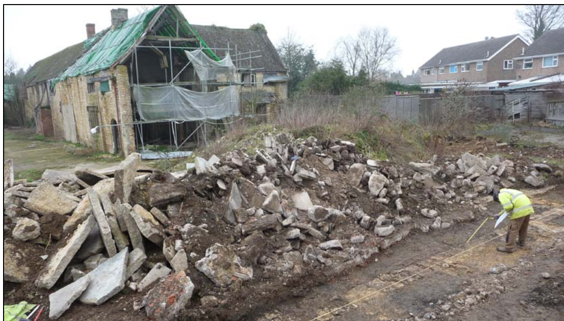
Figure 7: Trench 2; recording in progress; view north-west
