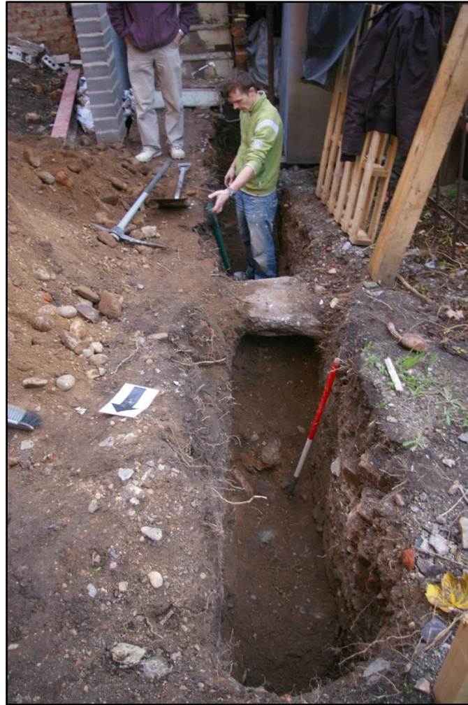
Plate 3: Extension foundation Trench 3 looking south-east
