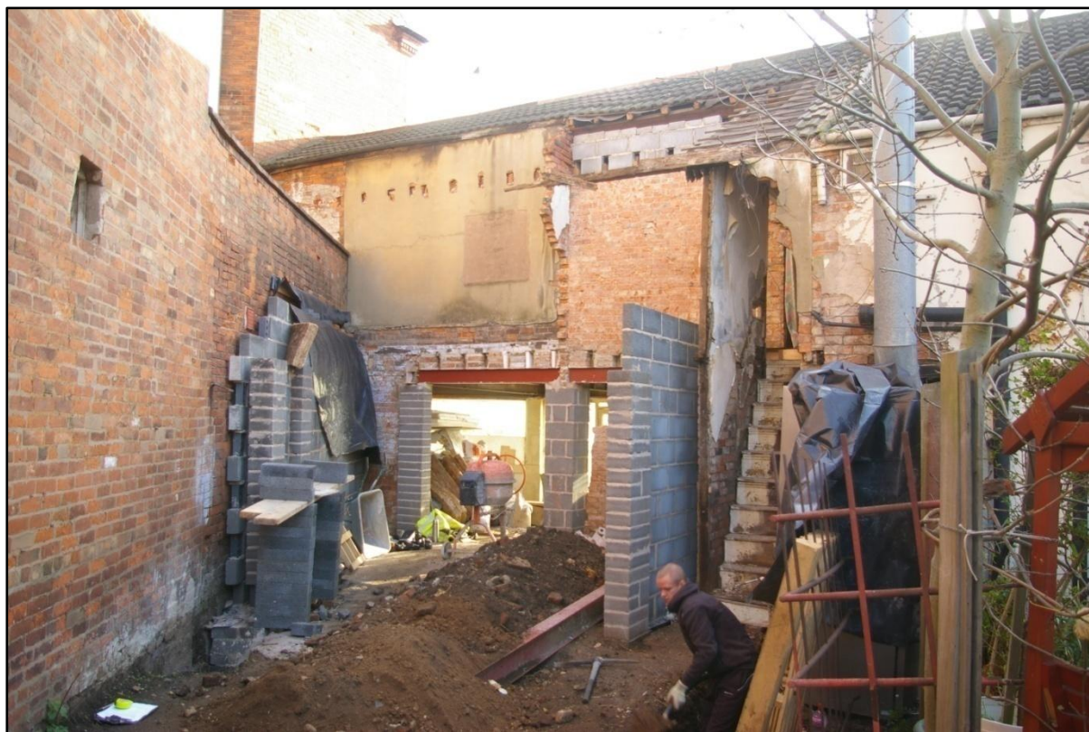
Plate 1: Development area at the rear of 29 Derby Square, Loughborough looking south-east
