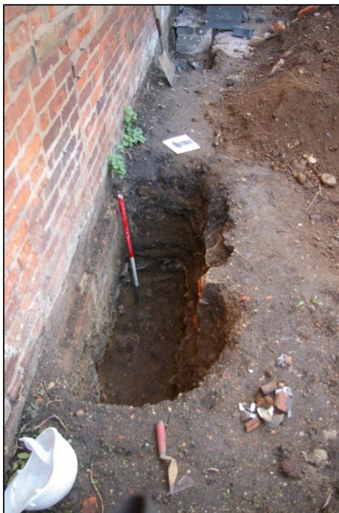
Plate 2: Extension foundation Trench 1 looking south-east
