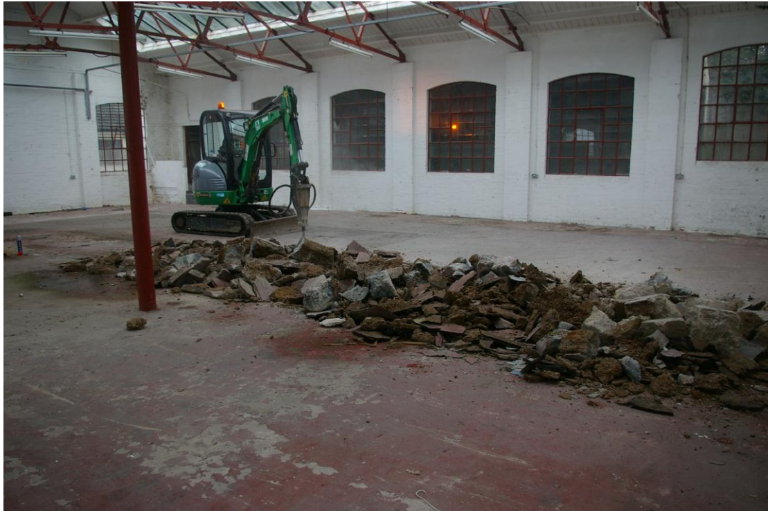
Plate 9: Concrete breaking in progress, Trench 3, looking west
