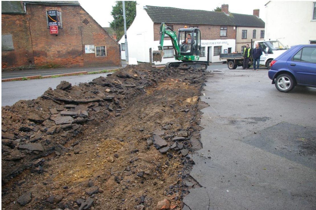
Plate 3: Removing asphalt on Trench 1, looking south
