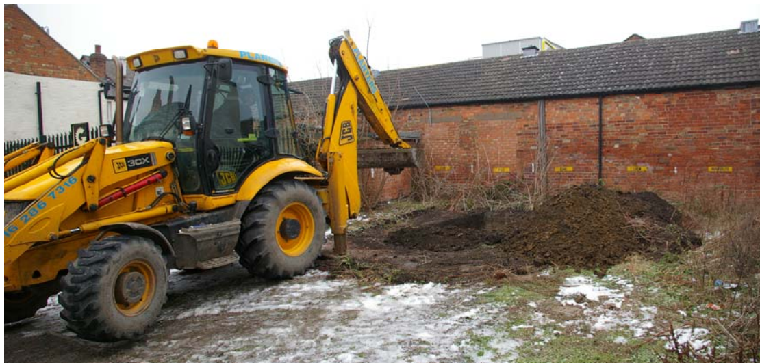
Plate 1: Work in progress, looking north-east
