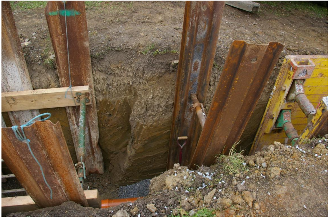
Plate 12: Sewer trench, looking west
