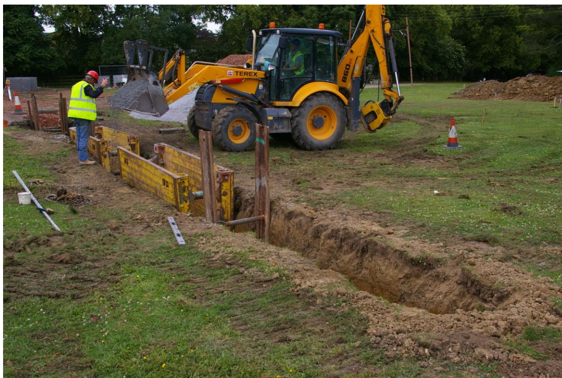
Plate 11: Work in progress on sewer trench, looking south south-west
