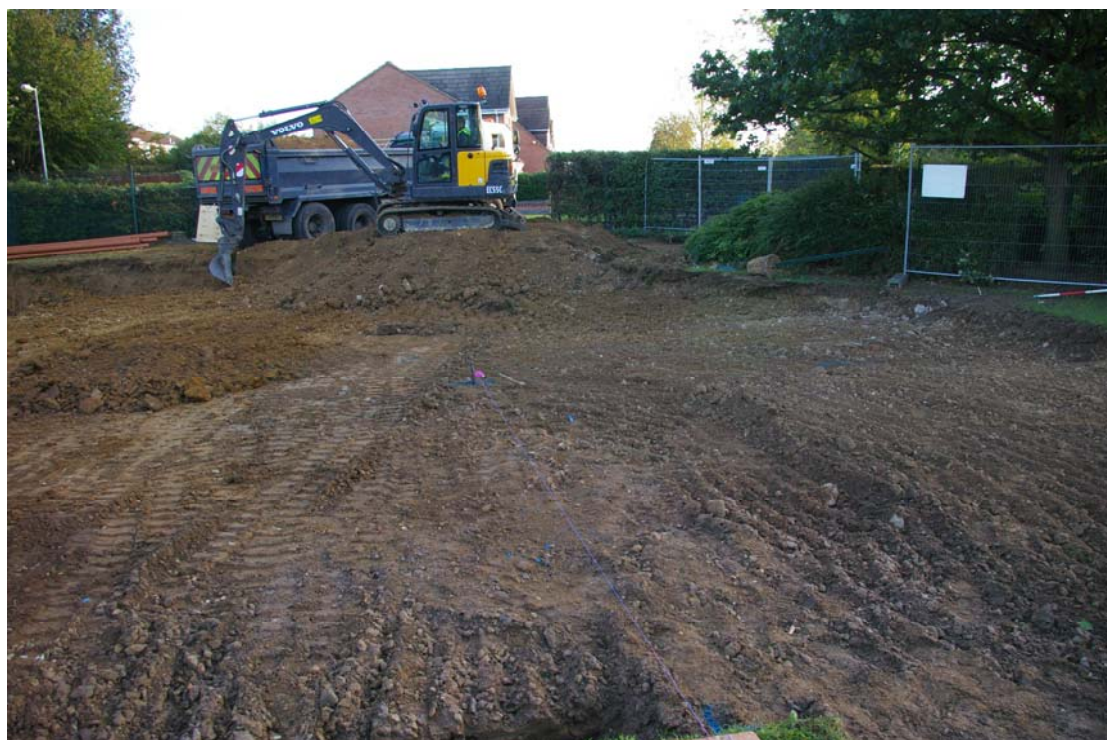
Plate 5: Most of area stripped, south-western end looking east
