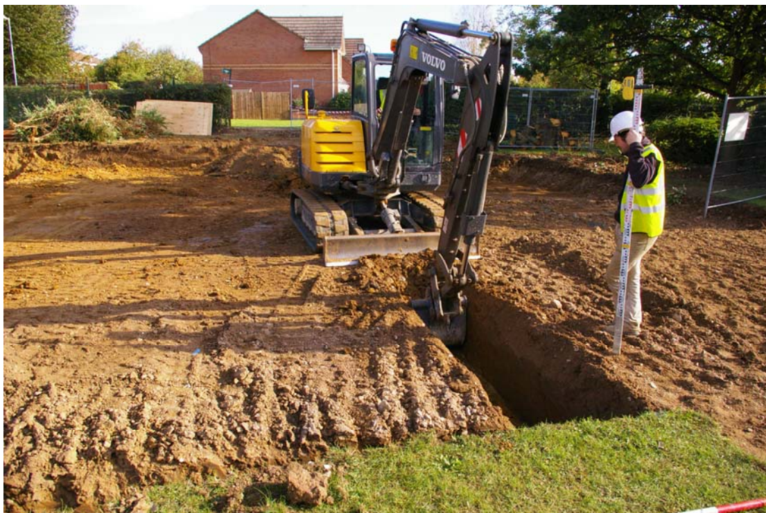
Plate 9: Work in progress on south-western trench, looking east
