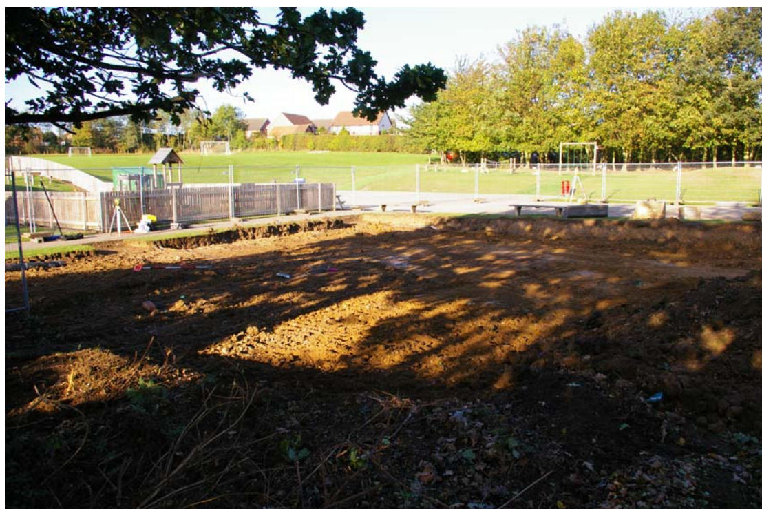
Plate 6: Area stripped looking north-west
