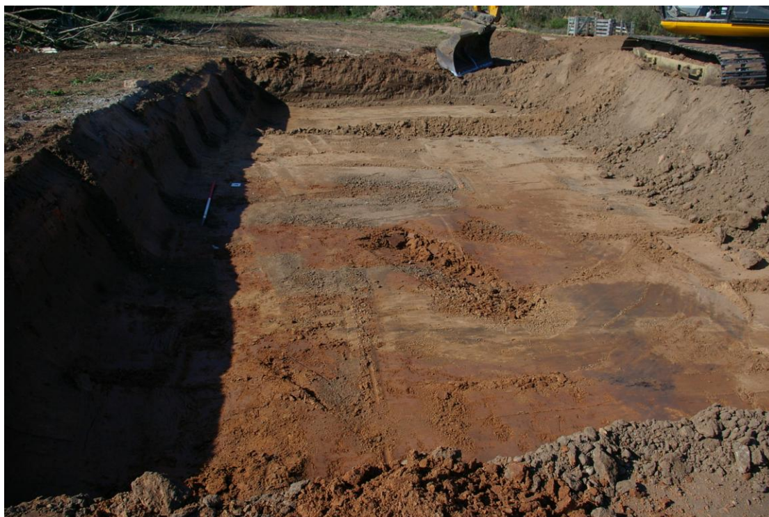
Plate 19: Stripped manège area, looking north-west
