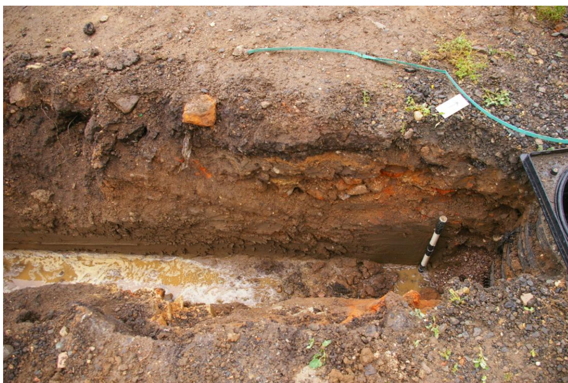
Plate 12: Northern end of drain trench, looking north north-west
