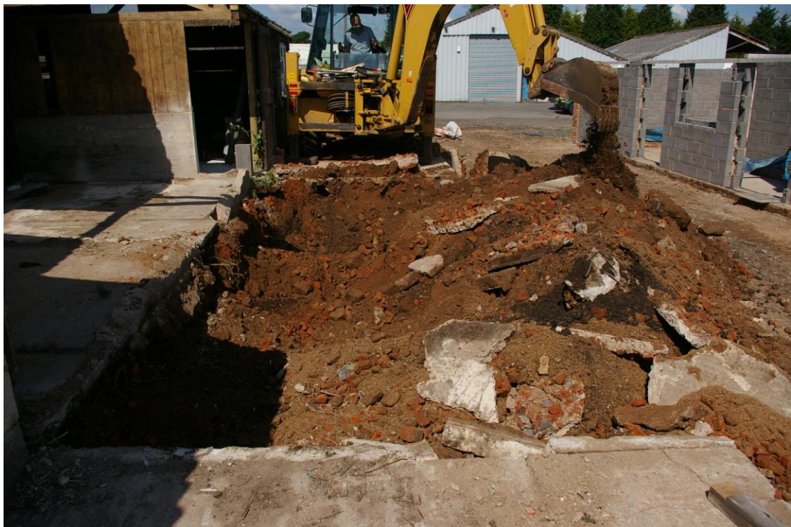
Plate 6: Work in progress on centre barns, looking west
