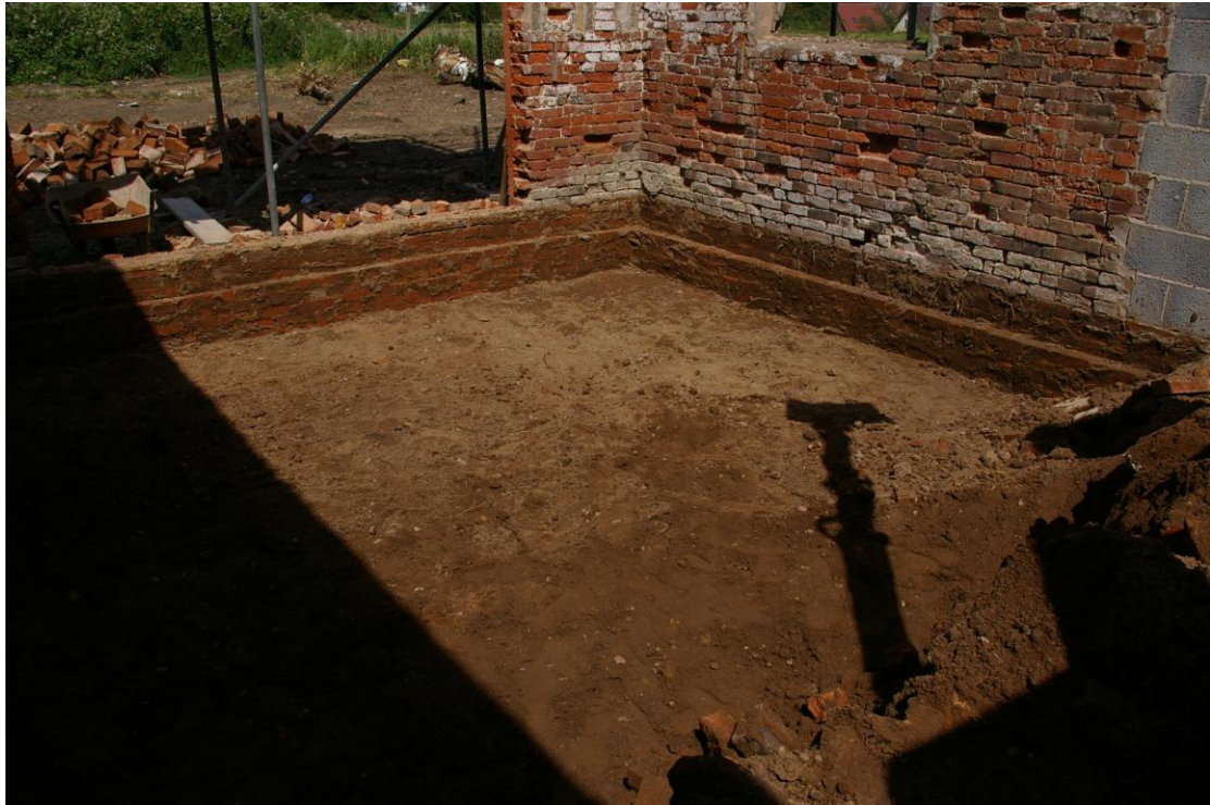
Plate 5: Floor fully excavated, looking north-east
