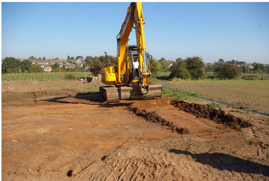
Plate 18: Work in progress on manège area, looking north
