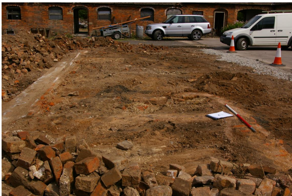
Plate 9: Concrete beam and brick foundations, looking east to two story range
