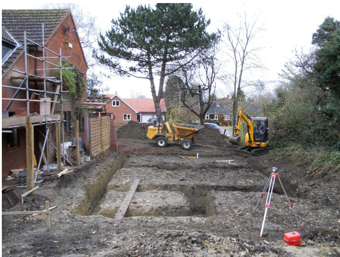
Figure 6. Excavated foundation trenches Looking east
