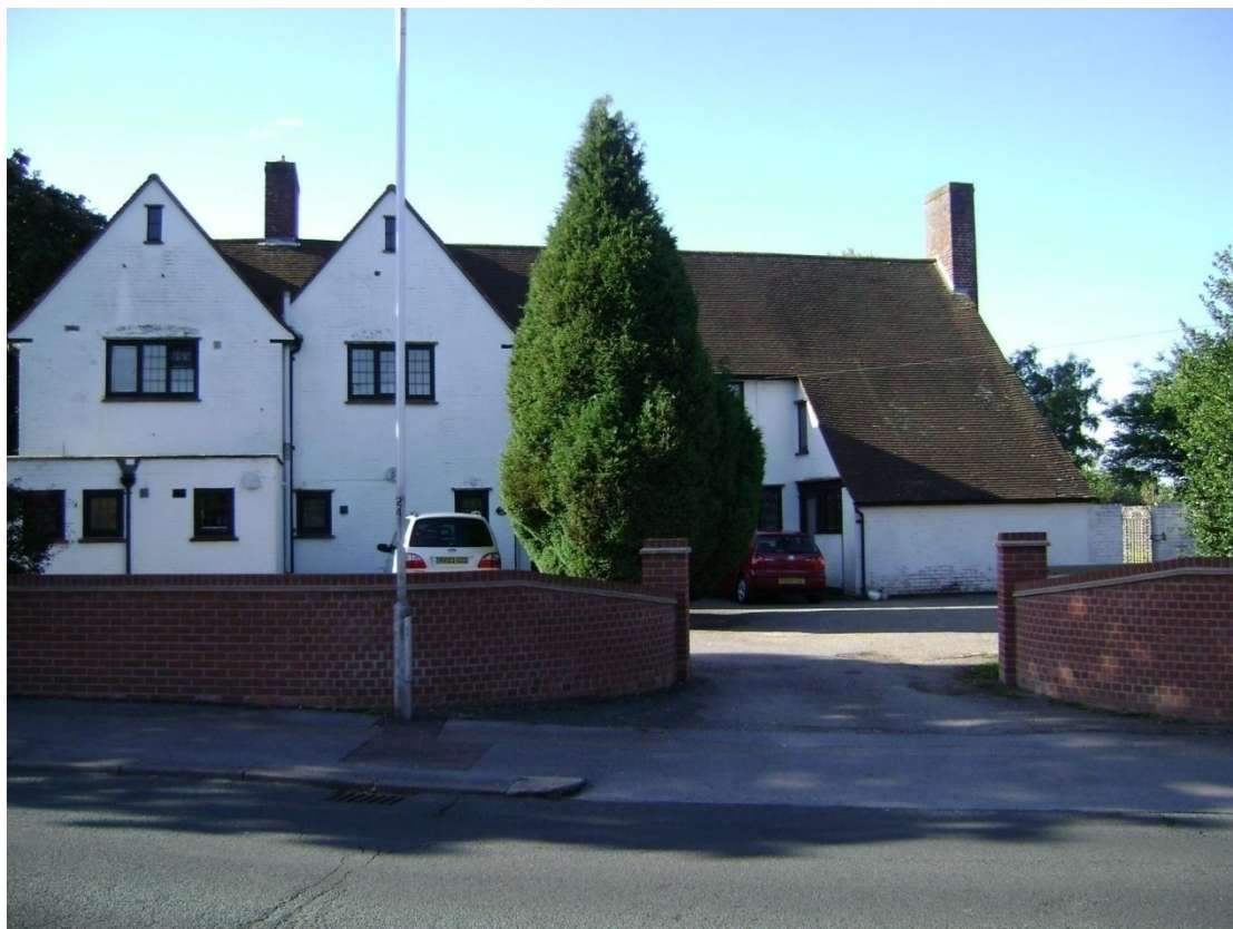
Figure 3. White Barn, 45 Cressingham Road Looking south. Photograph taken before commencement of work.
