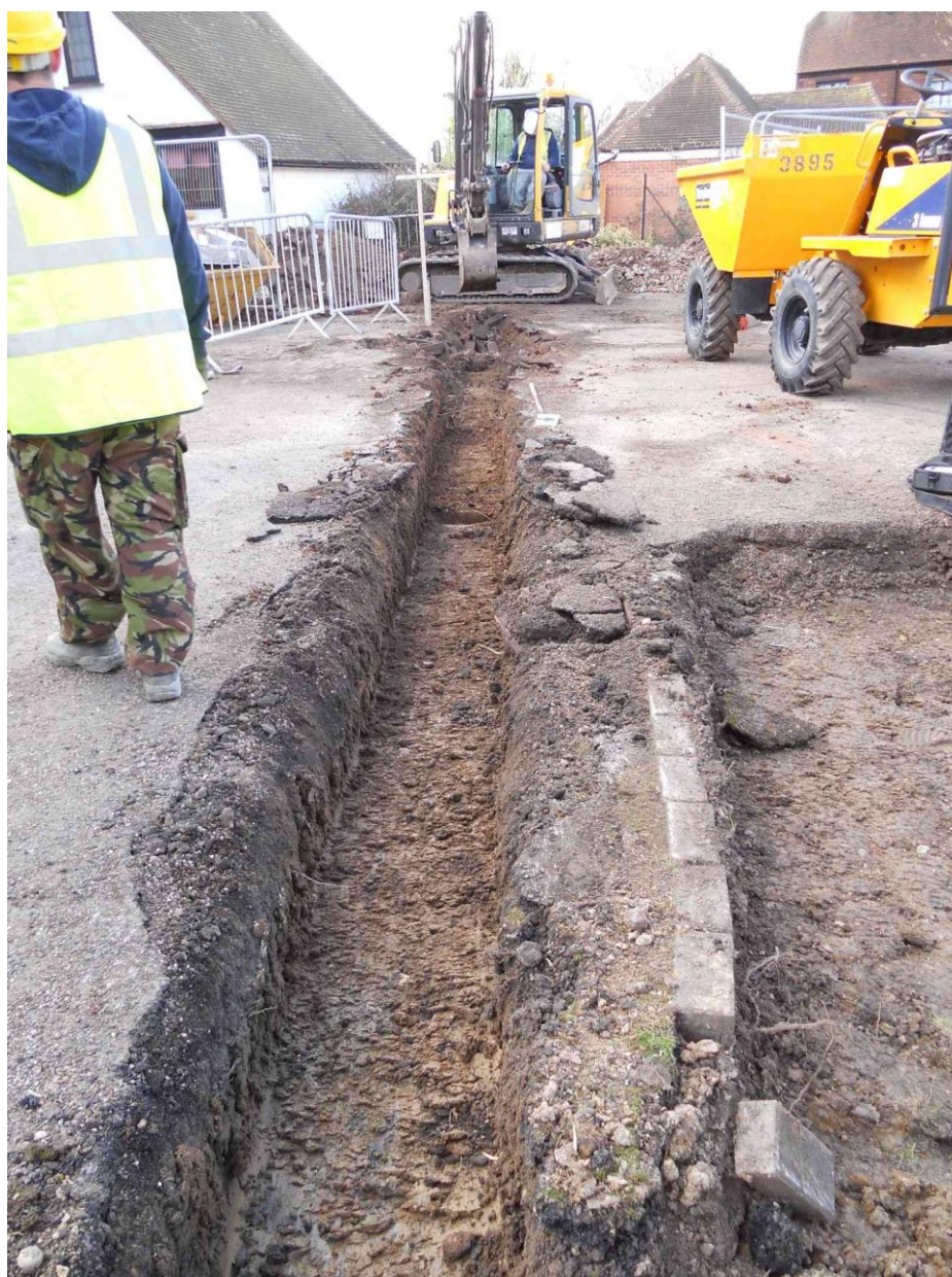
Figure 8. Service Trench Looking south-west. 1m scale
