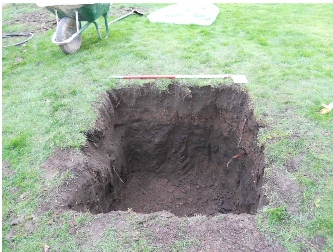
Figure 8. Soakaway, south facing section Looking north. 1m scale
