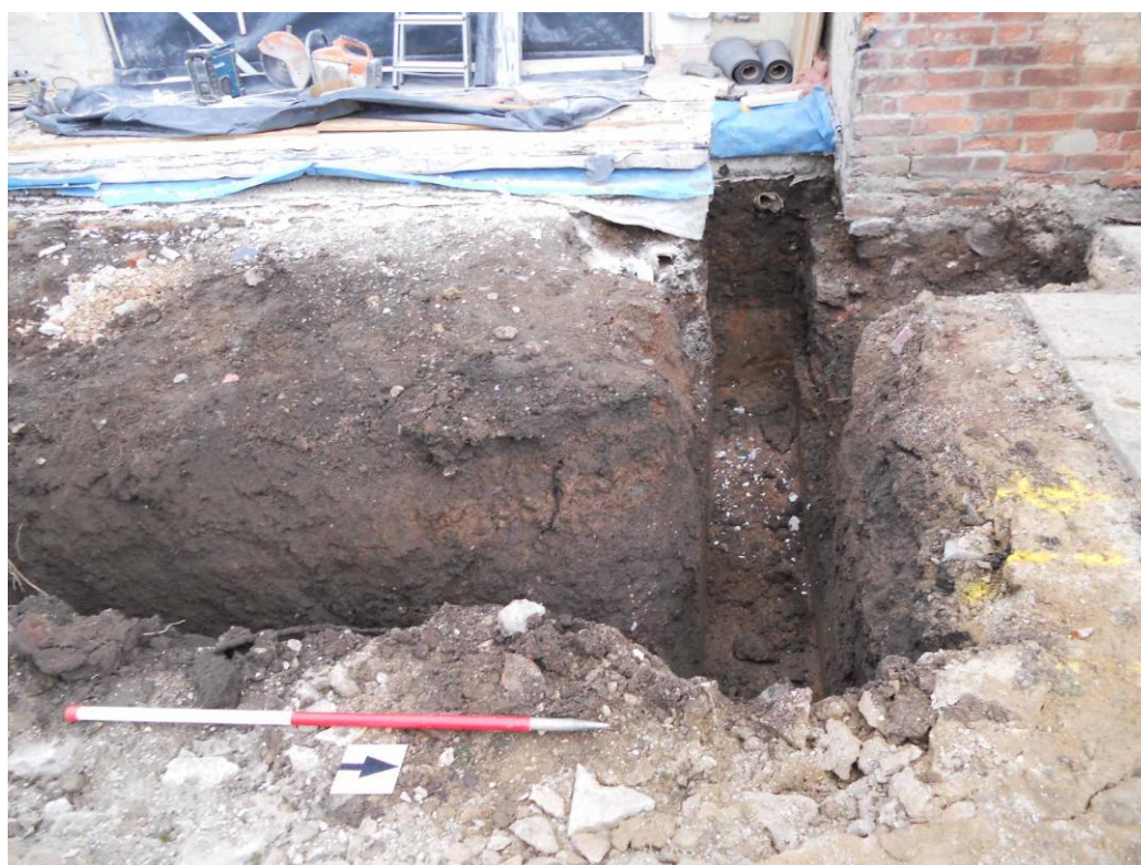
Figure 6. North arm of foundation trench Looking west. 1m scale
