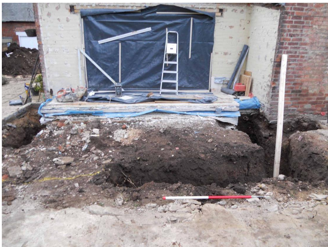
Figure 7. Foundation trench Looking west. 1m scale
