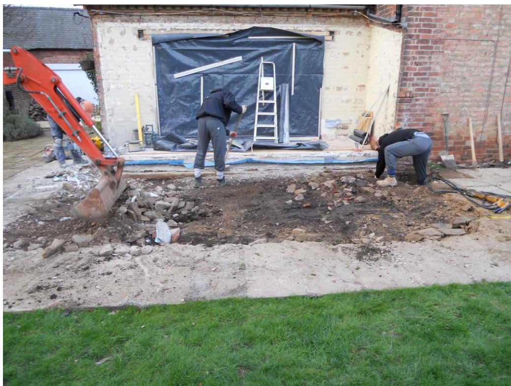
Figure 5. Ground reduction within footprint of new orangery Looking west
